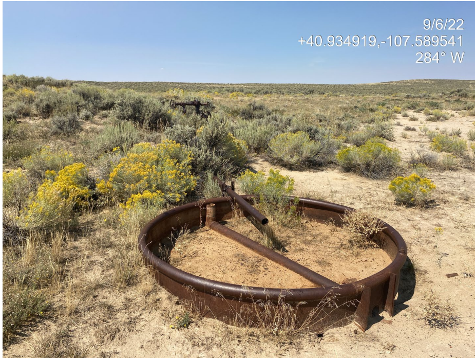
Photo 1. Photo shows where a pipe appears to have previously connected from the wellhead to a presently non-functioning tank.
