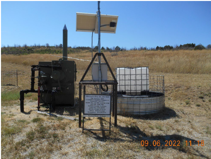
Separator. Secondary containment of chemicals
