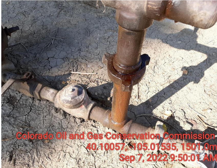
Photo 3 mechanical issue 2" flow line leaking around hammer union
