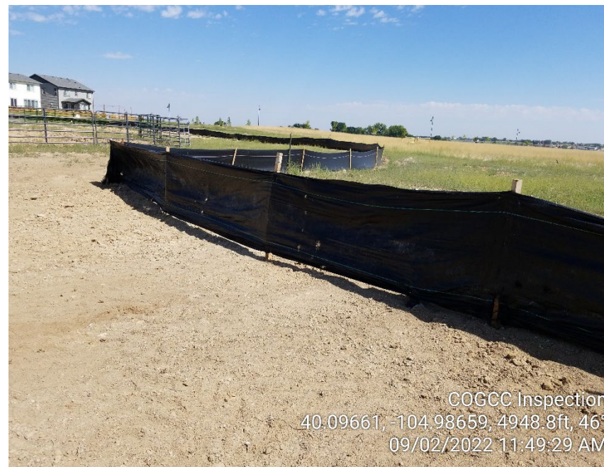
Photo 12 – Silt fence is inadequately installed
