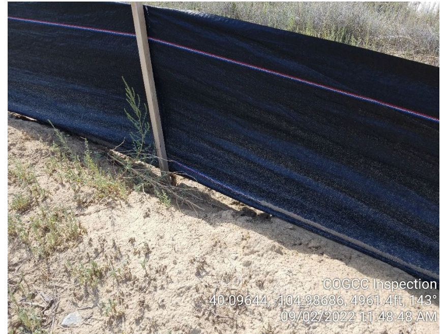
Photo 10 – Silt fence is inadequately installed
