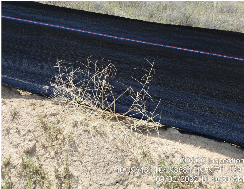
Photo 9 – Silt fence is inadequately installed
