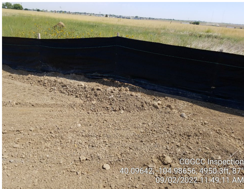
Photo 13 – Silt fence is inadequately installed
