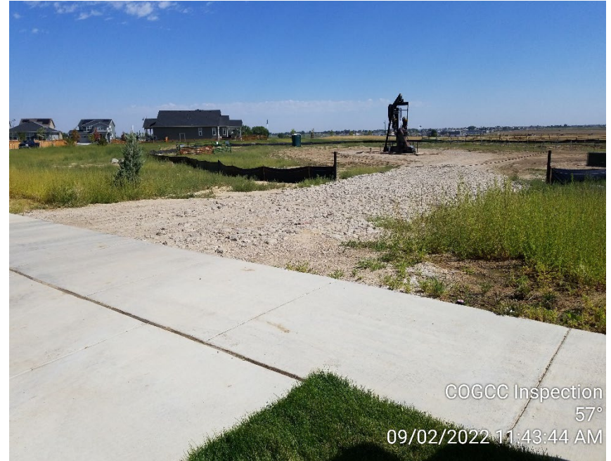
Photo 4 – Dirt being tracked off location observed in previous inspection has been cleaned. No maintenance appears to have been performed on vehicle tracking pad.
