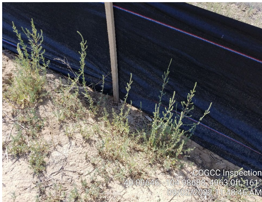
Photo 11 – Silt fence is inadequately installed
