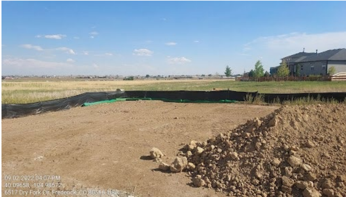
Photo 15 – Photo provided by KPK to COGCC documenting silt fence was repaired after COGCC left location.
