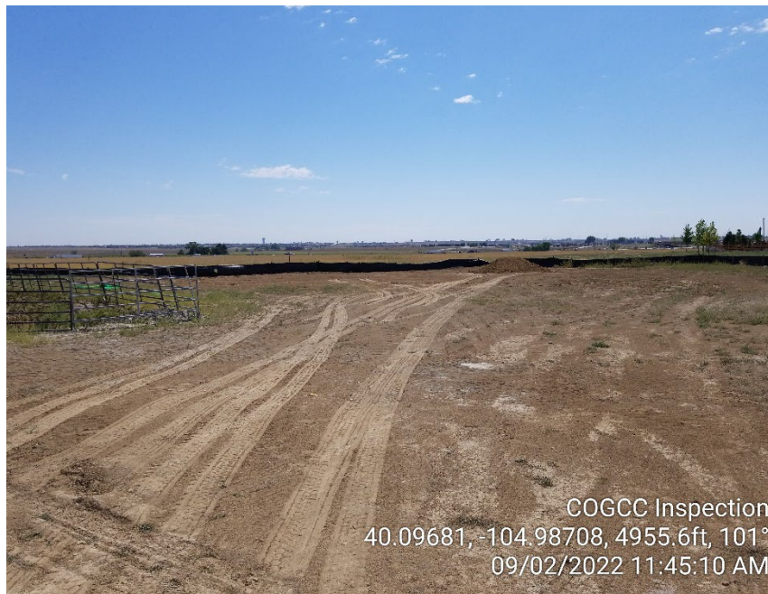
Photo 7 – Previously stored contaminated soil has been removed from location. One pile of soil for backfill has been stored on site.
