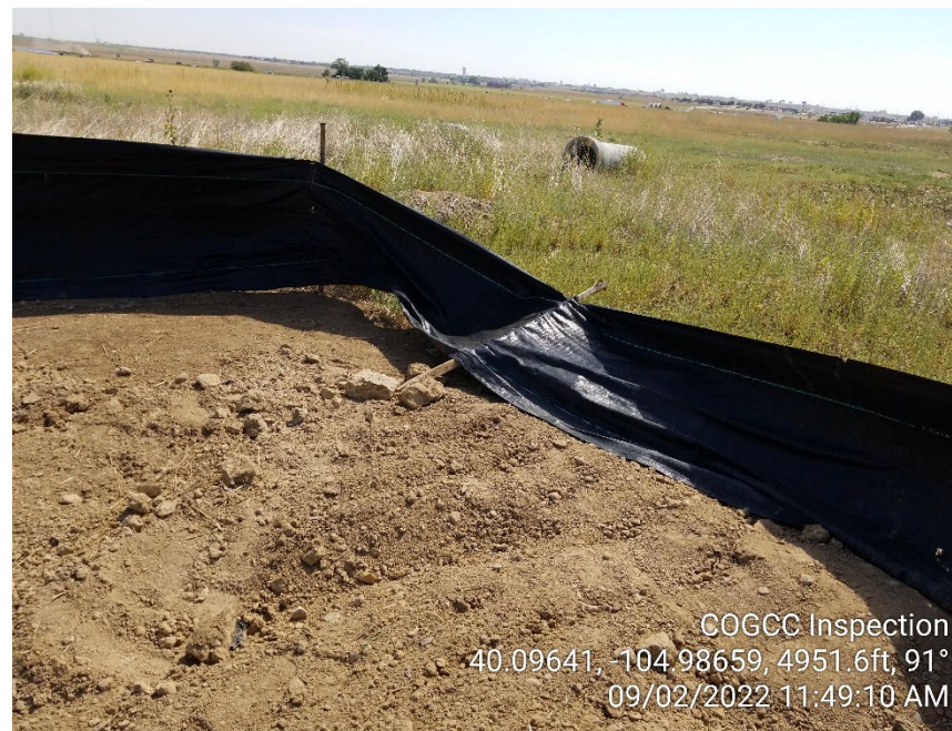
Photo 14 – Silt fence beginning to fall
