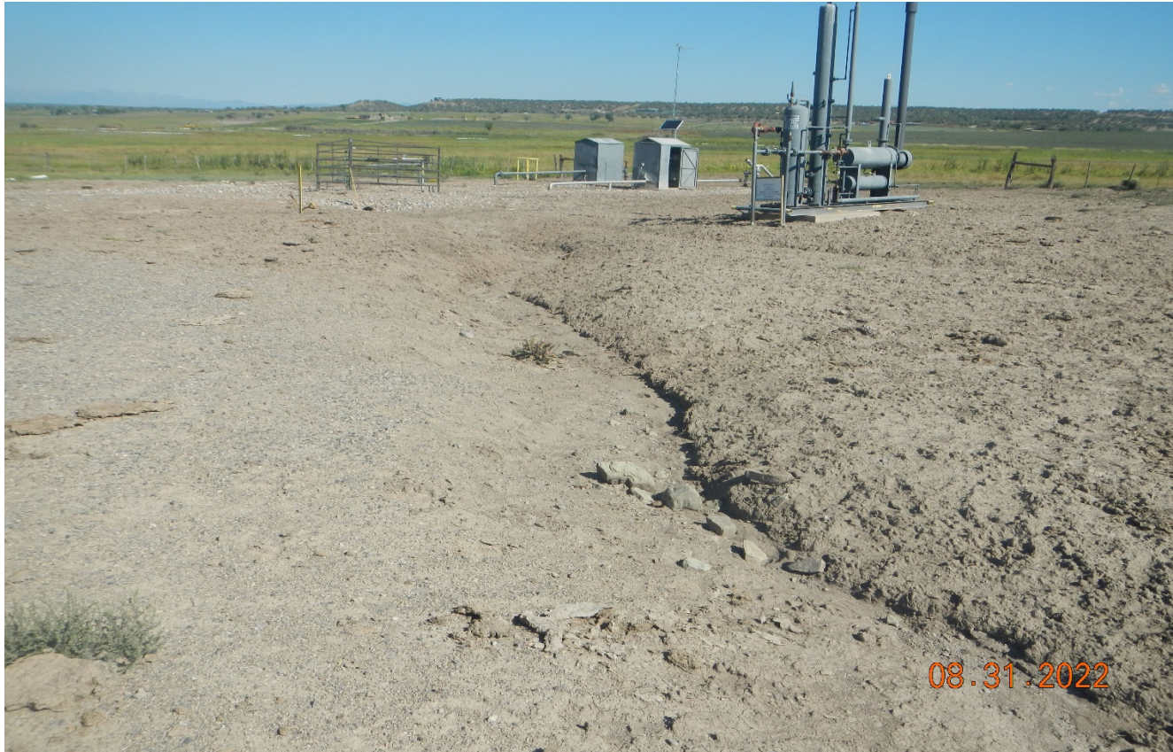
Photo 3. There is an erosion channel at the northeastern area of the location. BMP's need to be installed.
