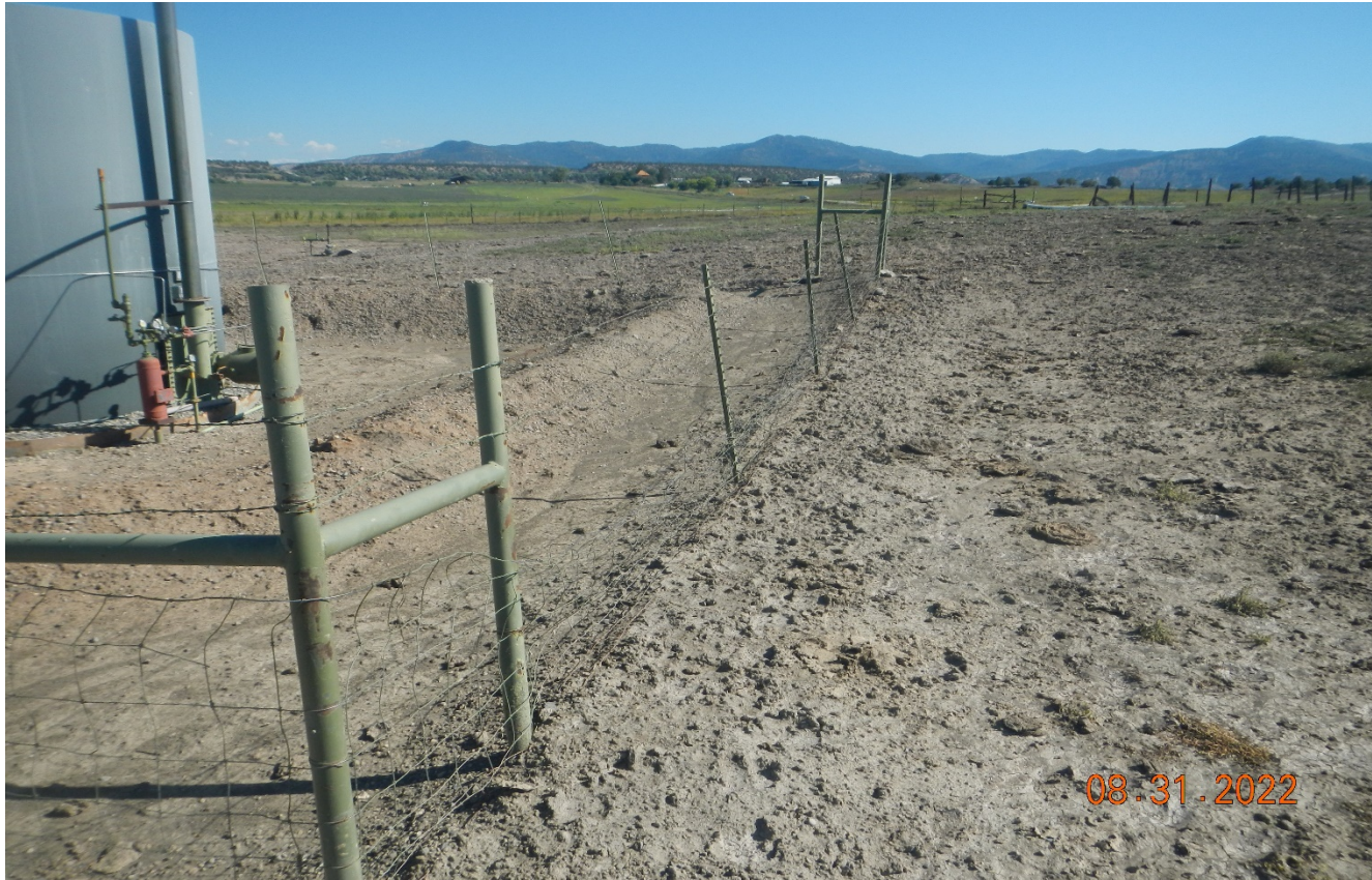
Photo 2. The fence around the tank battery is in need of maintenance to prevent livestock entry.
