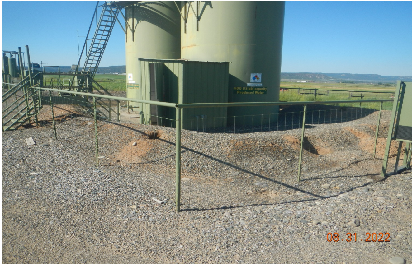
Photo 2. Facing toward the tank battery. There are animal holes in the berm which is compromising the containment.
