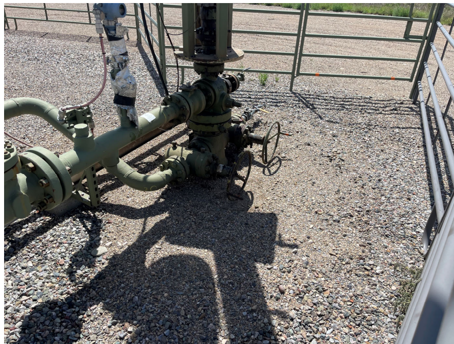
Lube oil stained soil at wellhead removed
