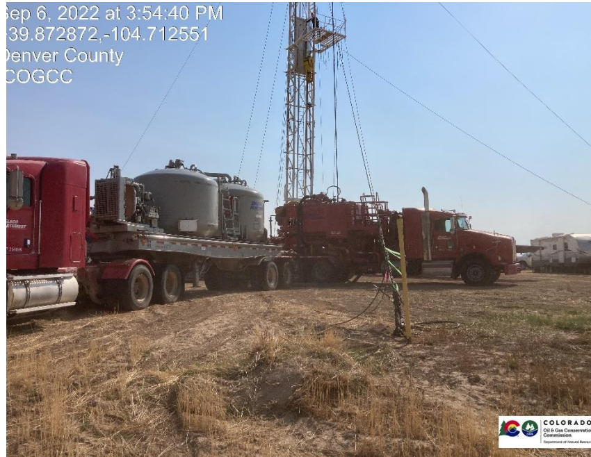
Pic 3 Cement truck
