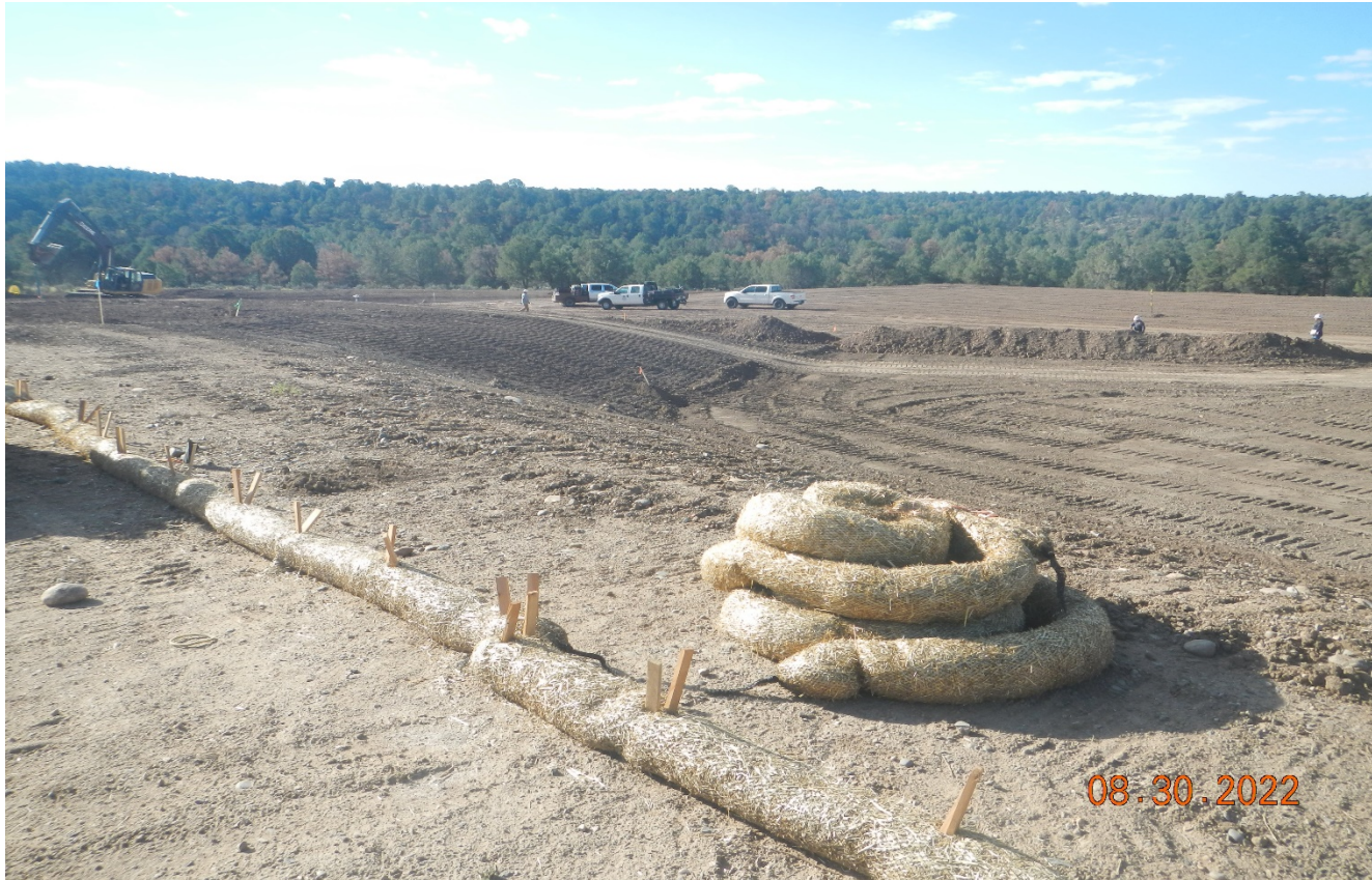
Photo 2. Facing southeast toward the location. The perimeter wattles shown in the photo were not trenched into the ground per good engineering practice.
