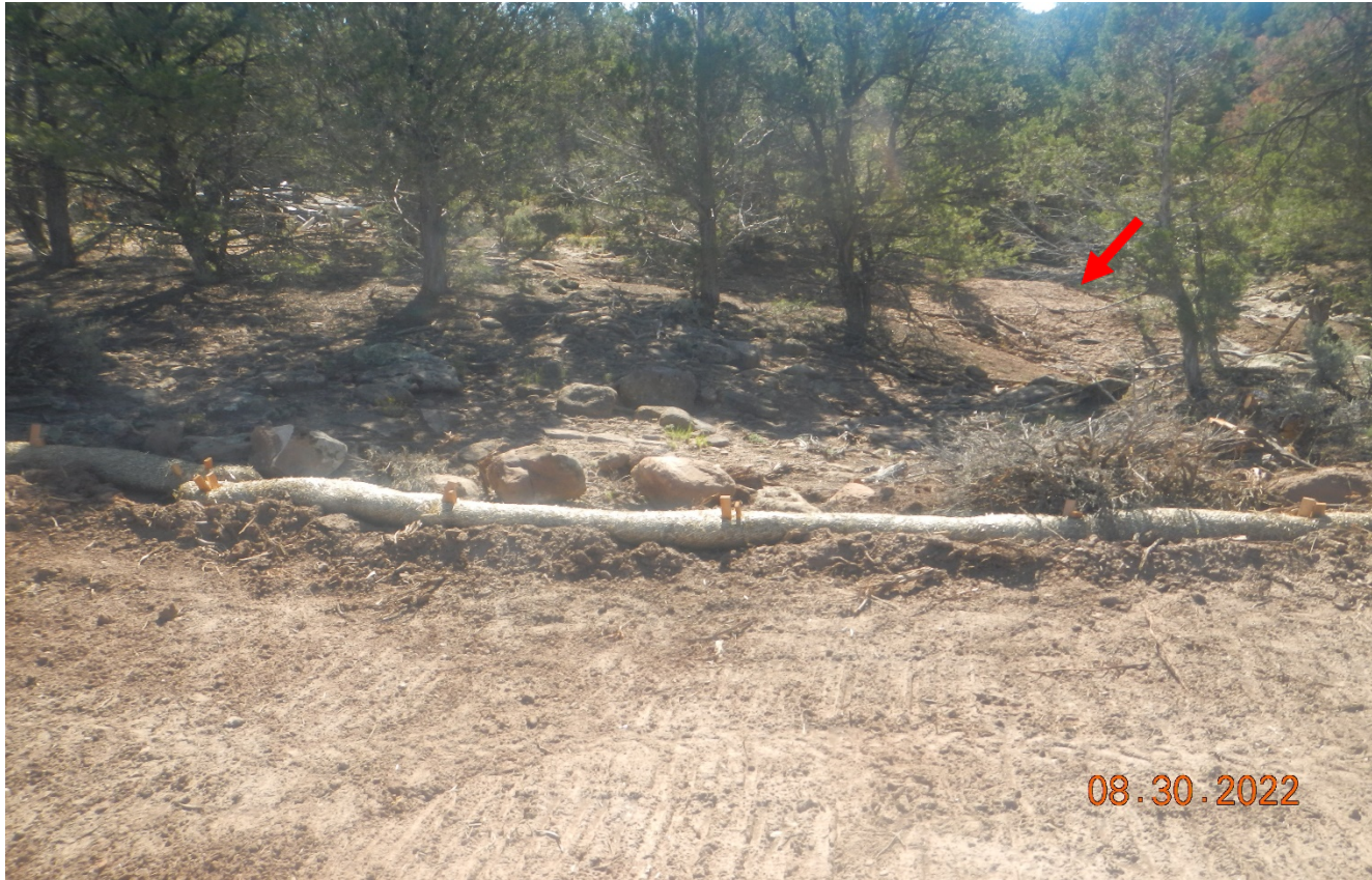
Photo 13. There is an ephemeral drainage show at red area approximately 60' from the wattles. The wattles installed will not prevent sediment migration offsite from the drainage shown at red arrow. Additional BMP's need to be installed which may include sediment trap, rip/rap ect. as determined and installed by good engineering practice.
