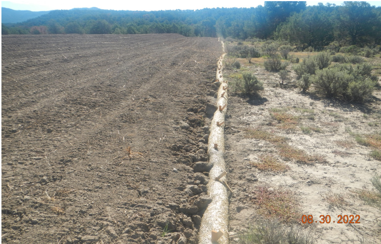
Photo 9. South side of the location facing southeast. There is soil piled up and overtopping the stormwater wattles. It appears the 6" wattles are insufficient size.
