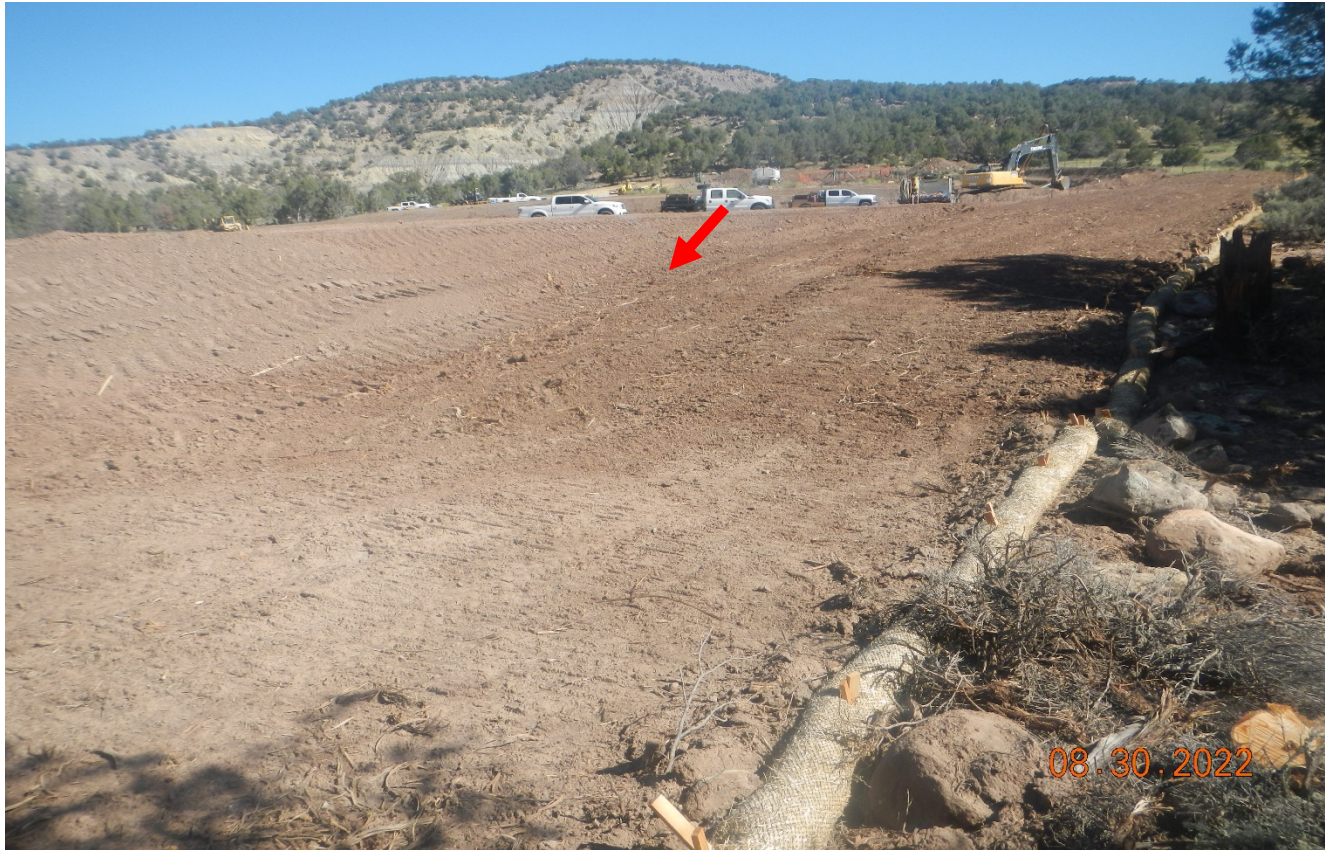
Photo 12. Southeast corner of the location facing north. There is insufficient BMP's installed in this area. The wattles installed will not prevent sediment migration offsite from the drainage shown at red arrow. Additional BMP's need to be installed which may include sediment trap, rip/rap ect. as determined and installed by good engineering practice.
