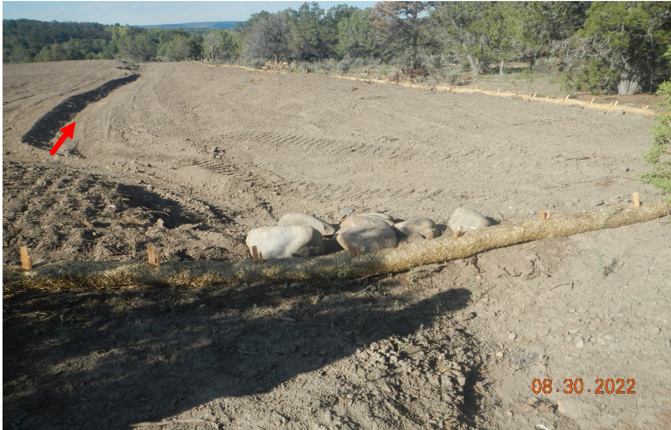
Photo 4. Facing southwest at the west side of the location. The rock inlet protection is insufficient in this area. Additional rock needs to be installed in this area and should include angular rock and geotextile. Additionally the stormwater drainage shown at red arrow consists of loose soil with no BMP's to prevent erosion.
