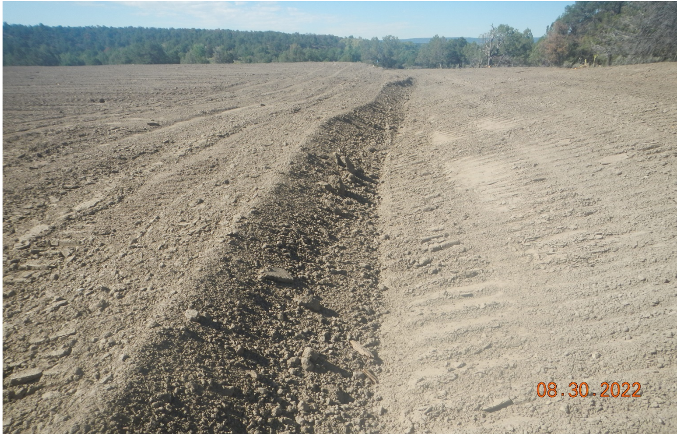
Photo 5. Facing southwest toward the stormwater diversion berm. The berm shown on the left is not compacted and loose soils are susceptible to erosion. The topsoil pile on the right side should be separated from the pad material.
