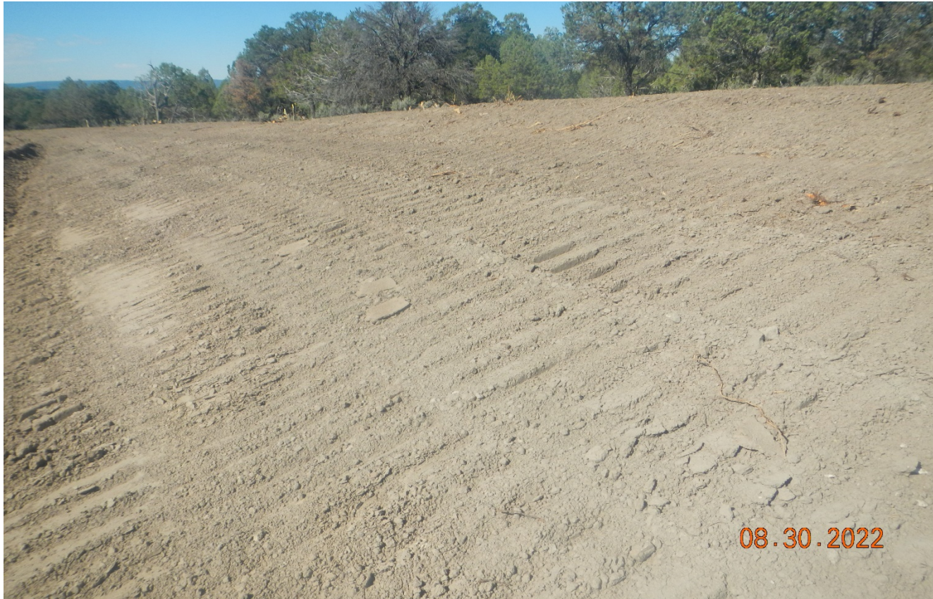
Photo 6. The topsoil pile is not properly tracked for temporary stabilization. Tracking must be performed perpendicular to the slope.
