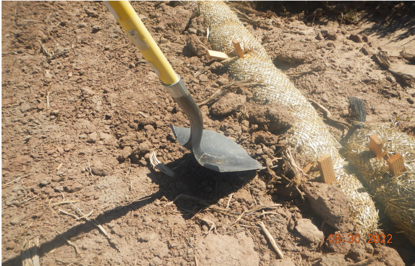
Photo 10. There is soil piled up and overtopping the stormwater wattles. It appears the 6" wattles are insufficient size.
