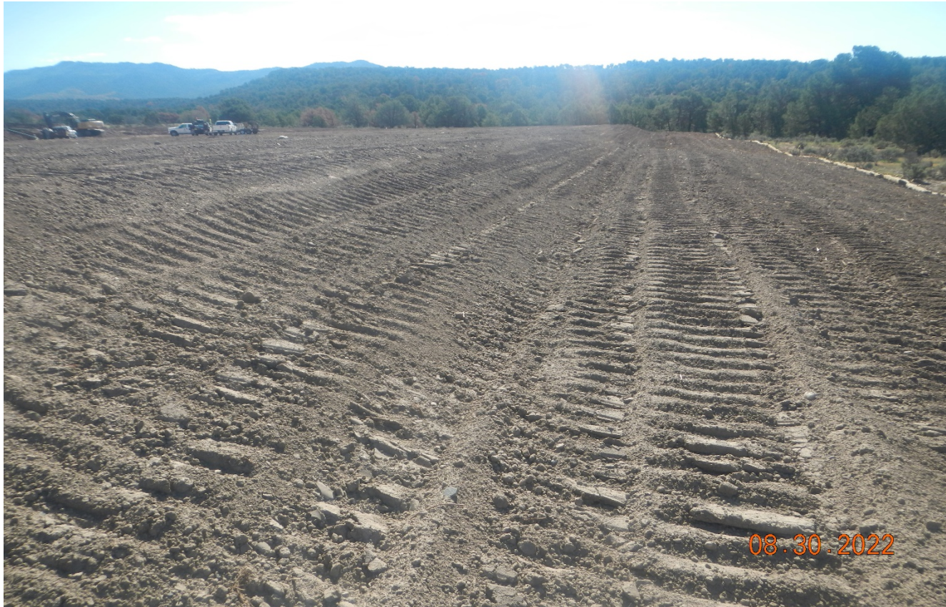
Photo 8. Facing southeast along the fill slope of the location. Tracking was not performed perpendicular to the slope.
