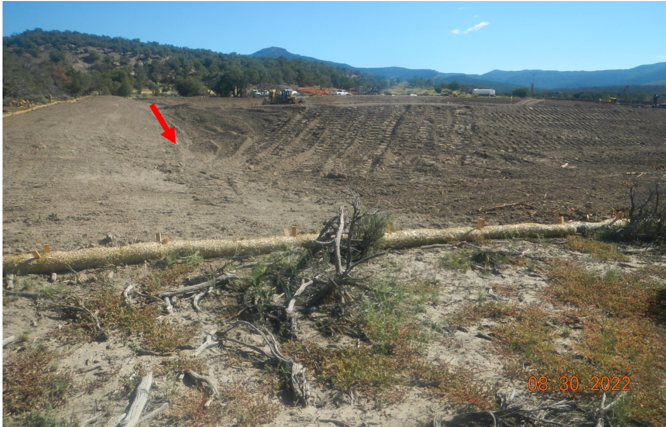
Photo 7. Southwest corner of the location facing northeast. There is insufficient BMP's installed in this area. The wattles installed will not prevent sediment migration offsite from the drainage shown at red arrow. Additional BMP's need to be installed which may include sediment trap, rip/rap ect. as determined and installed by good engineering practice.
