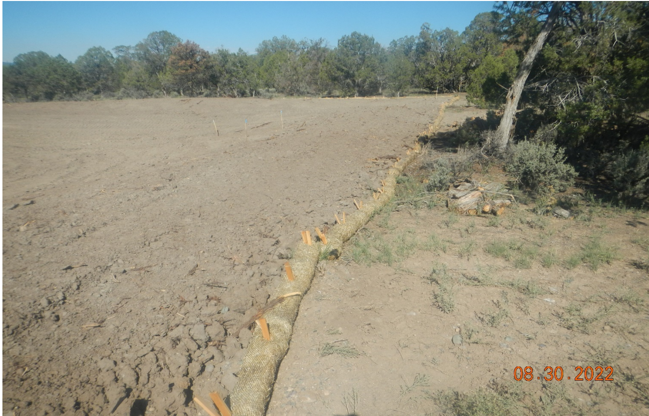
Photo 3. Facing toward the northwest side of the location. There is soil pile up and overtopping the stormwater wattles. It appears the 6" wattles are insufficient size.
