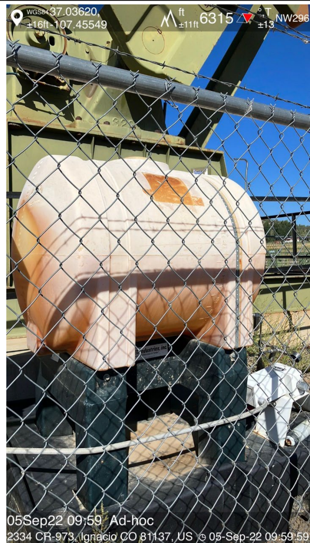
IMG 08 Chemical tank with no label/sign
