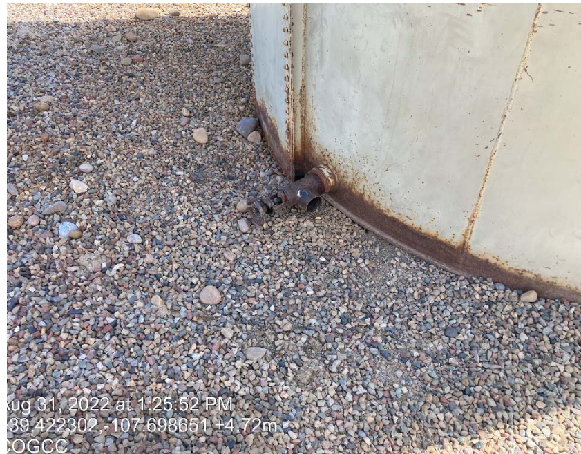
Valve missing cap/plug
