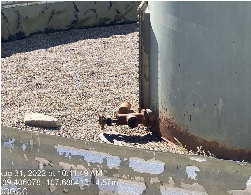
Valve missing cap/plug
