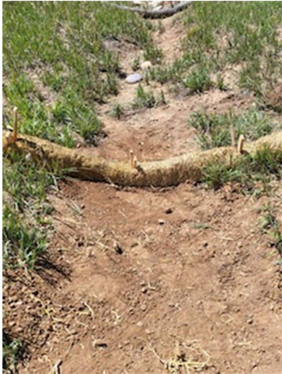
Replaced older wattles with new ones and reset existing wattles that were in good condition
