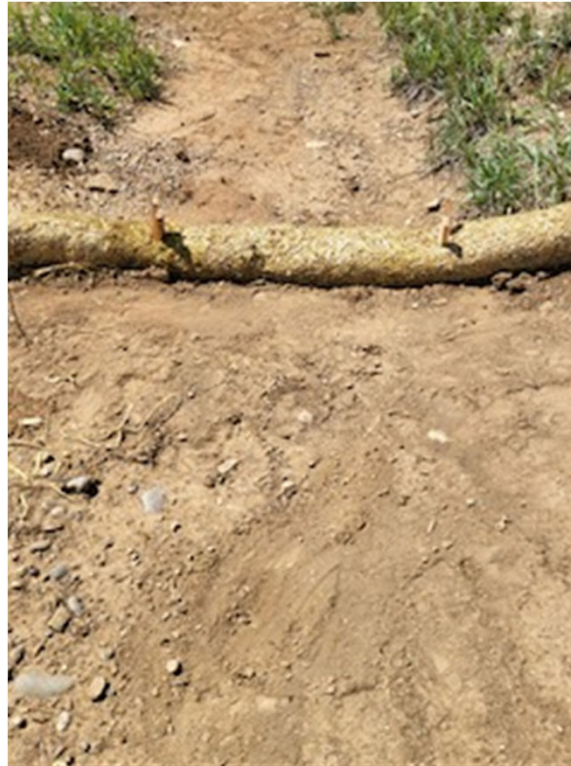
Replaced older wattles with new ones and reset existing wattles that were in good condition
