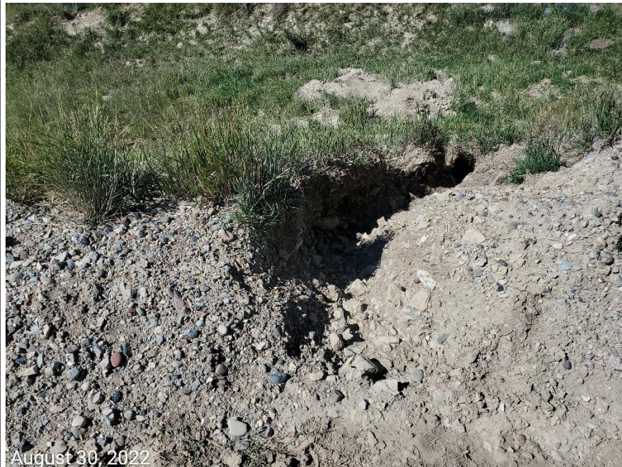
Photo 4: Photo taken from the sediment trap on the southwest end of the Location; BMP has not been maintained in proper functioning condition; photo shows gully erosion and degradation to the control.
