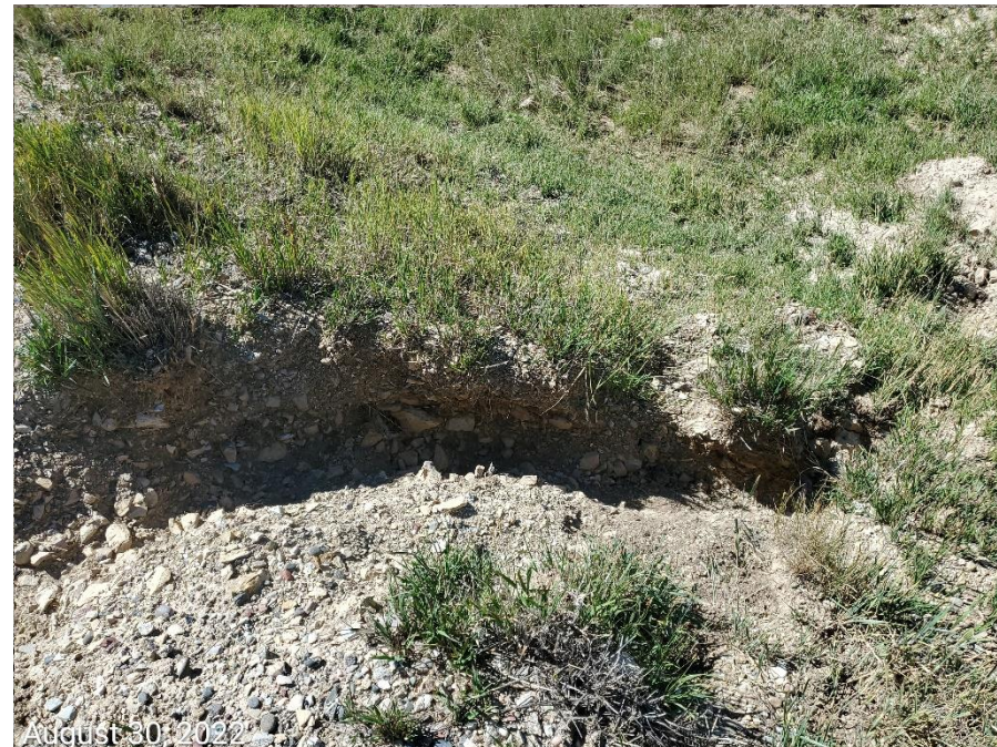
Photo 4: Photo taken from the sediment trap on the southwest end of the Location; BMP has not been maintained in proper functioning condition; photo shows gully erosion and degradation to the control.
