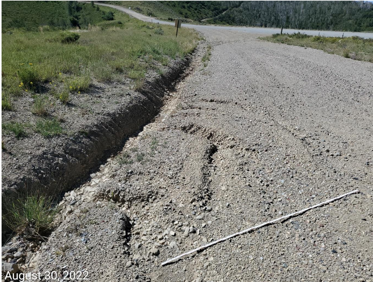
Photo 6: Photo taken from the access road, facing south. Photo shows stormwater runoff from the Location has resulted in erosion degradation at the Location entrance, and the access road; required stormwater and erosion control measures pursuant to Rule 1002.f remain missing or insufficient. 6 foot measuring stick for reference.
