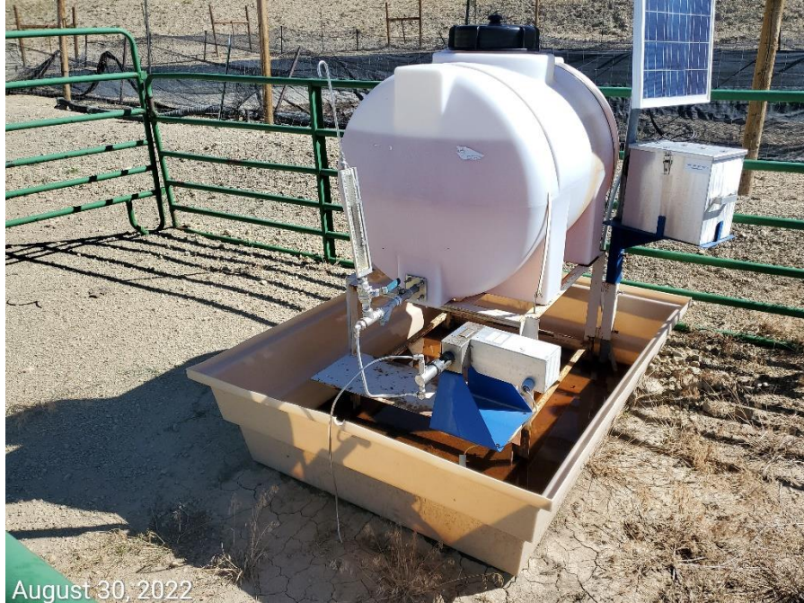
Photo 3: Photos show wildlife protection devices at the two methanol tanks on the Location remain missing or insufficient.
