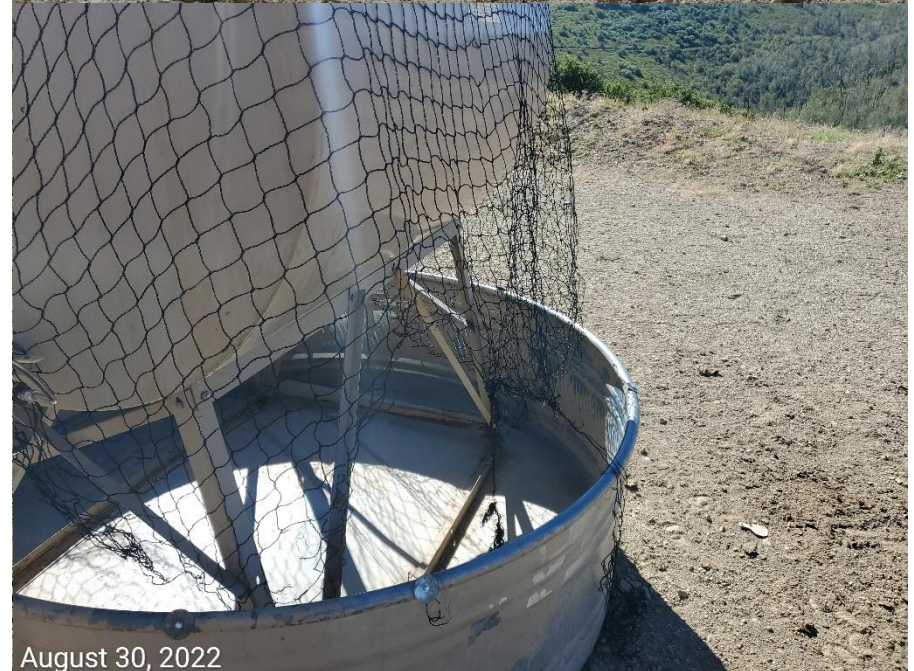
Photo 3: Photos show wildlife protection devices at the two methanol tanks on the Location remain missing or insufficient.
