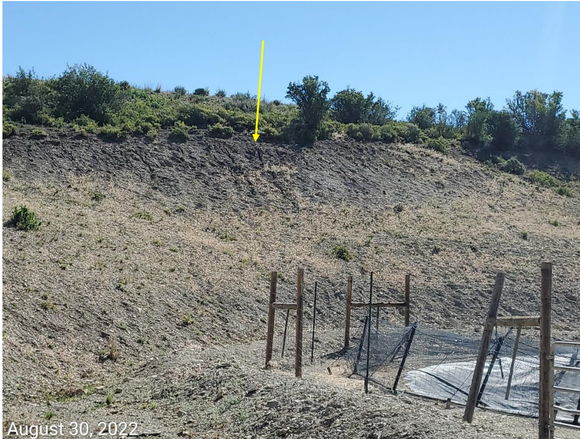
Photo 5: Photo shows erosion degradation on the cut slopes; stormwater and erosion control BMPs remain missing or insufficient.
