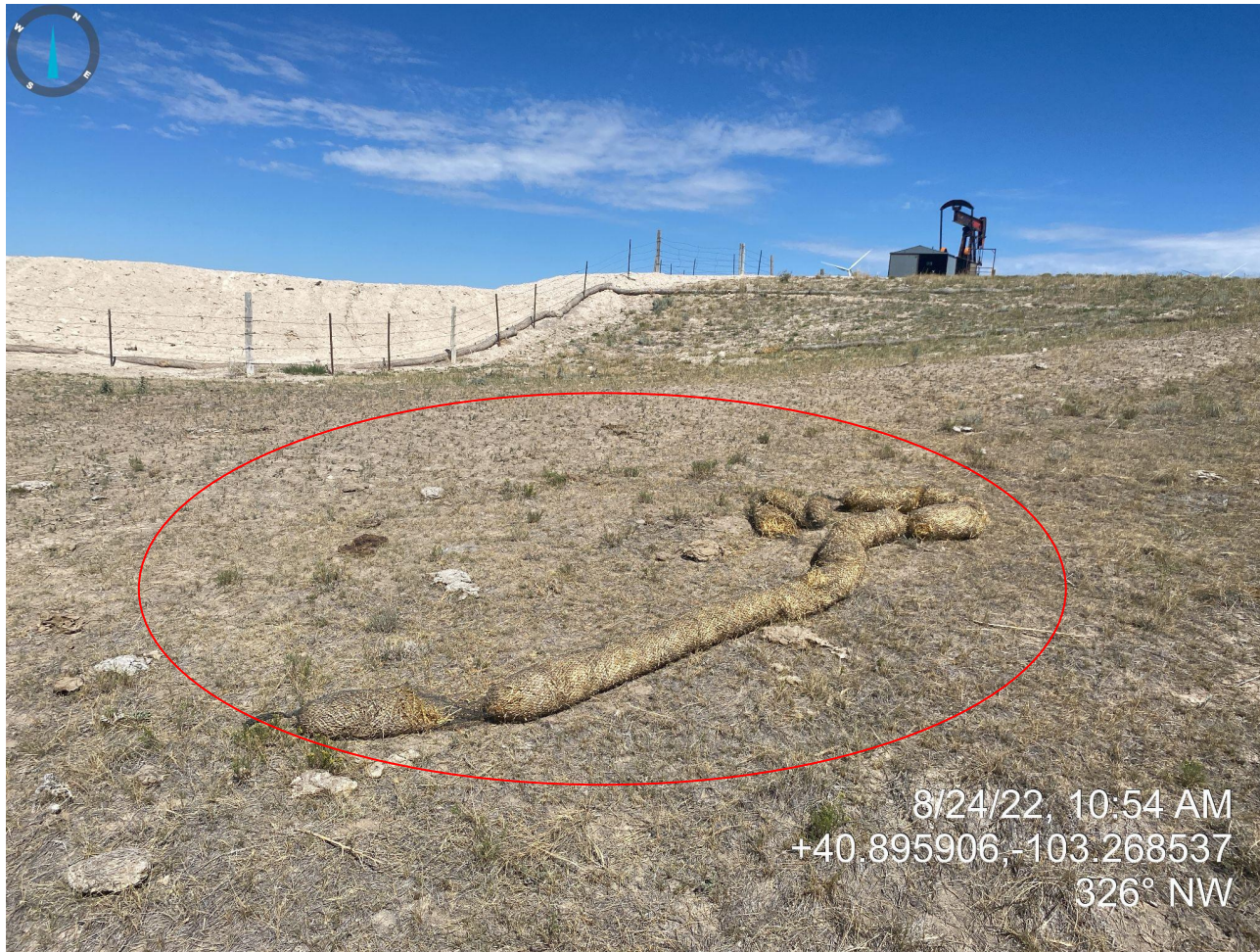
Photo 9. Photo taken southeast of location within salt kill area, facing northwest. Photo illustrates straw wattle was not properly installed and displaced within affected area; this is now considered debris and needs to be disposed of accordingly.
