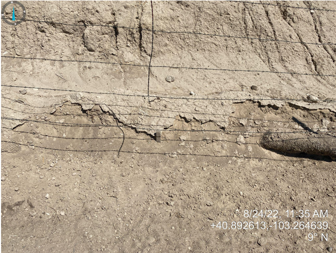
Photo 19. Close up photo illustrates missing straw wattle.
