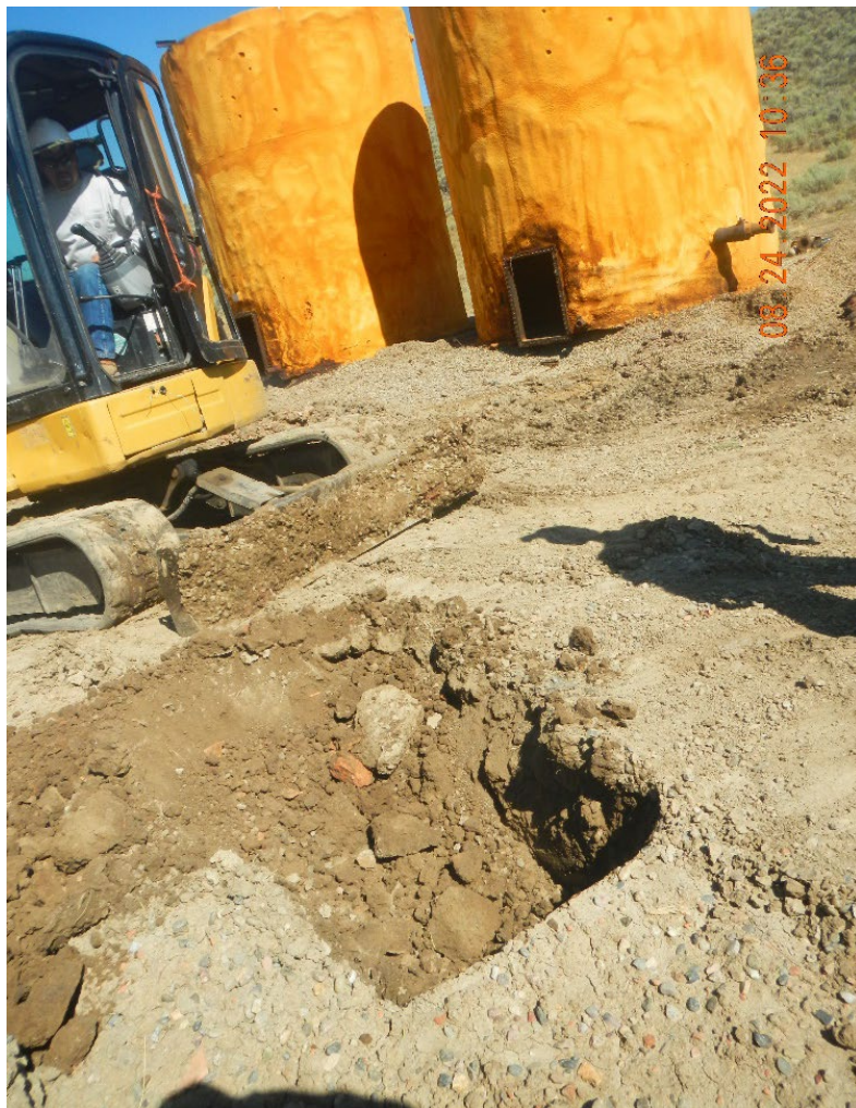
Photo #4 Sample at flowline from wellhead to tank battery. This was the only known flowing on the location. The flowline was removed from the ground.
