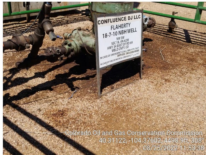
Photo 2 – 18-7-10 Wellhead – Stained Soil
