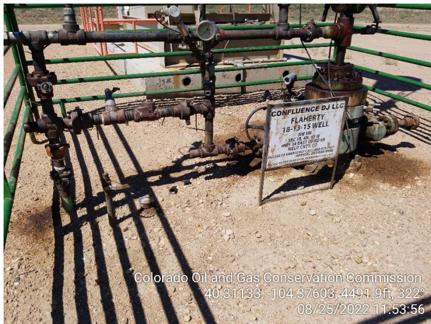
Photo 3 – 18-13-15 Wellhead – Stained Soil
