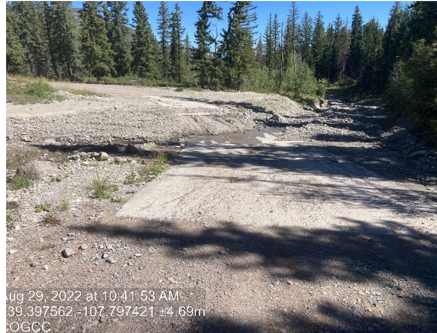
Access road at creek crossing washed out
