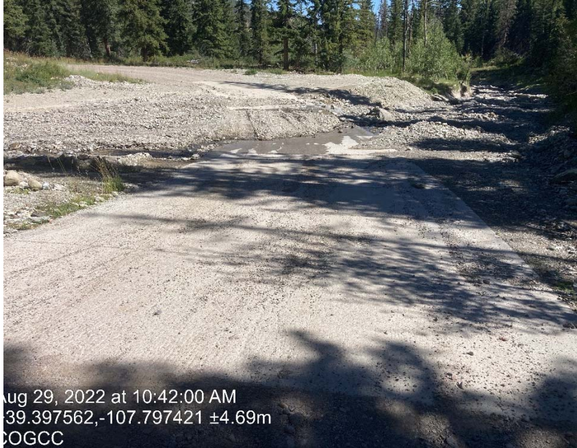
Access road at creek crossing washed out
