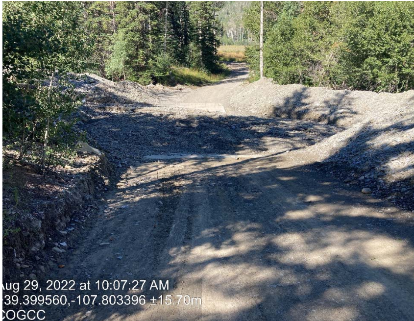
Access road at creek crossing washed out
