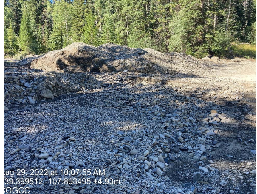
Access road at creek crossing washed out
