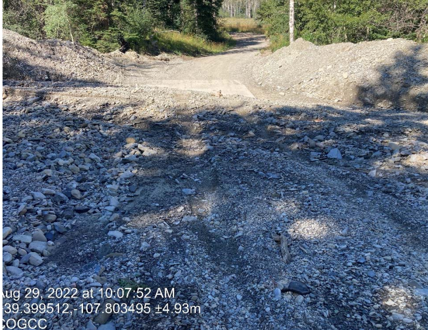
Access road at creek crossing washed out
