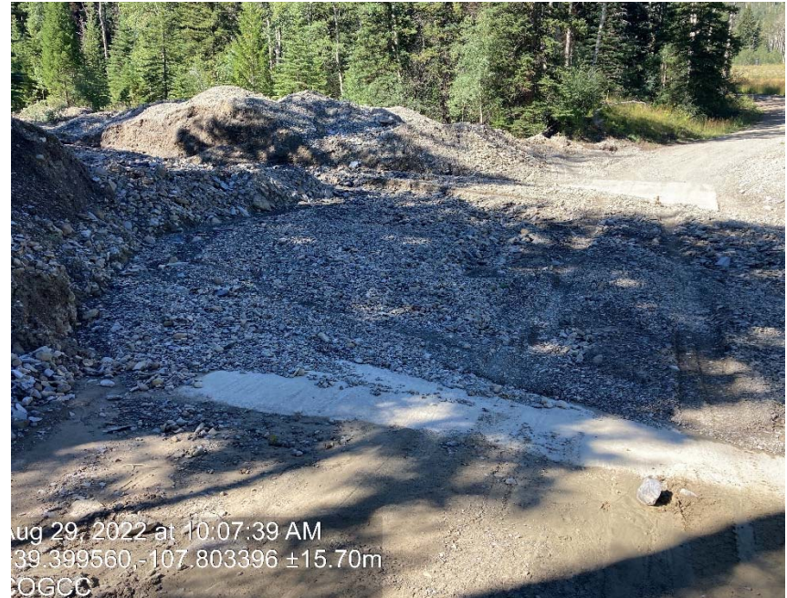
Access road at creek crossing washed out
