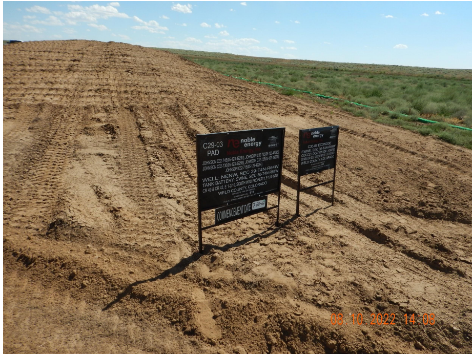
Photo 1. Photo taken from the northwestern location, facing South. Photo illustrates the Operator sign on the topsoil stockpile. Topsoil has been temporarily stabilized with equipment tracking.
