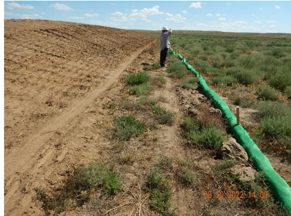
Photo 2. Photo taken from the western location, facing South. Photo illustrates filtrex has been installed around the entire perimeter of location.
