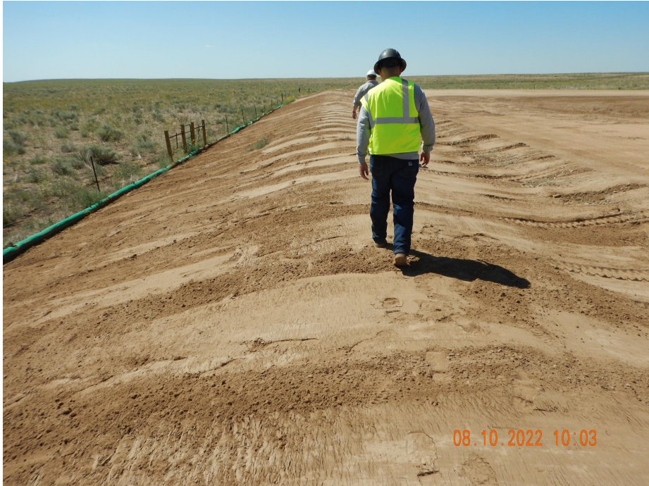
Photo 5. Photo taken from the eastern location, facing South. Photo illustrates a swale area that is directed to the sediment basin.
