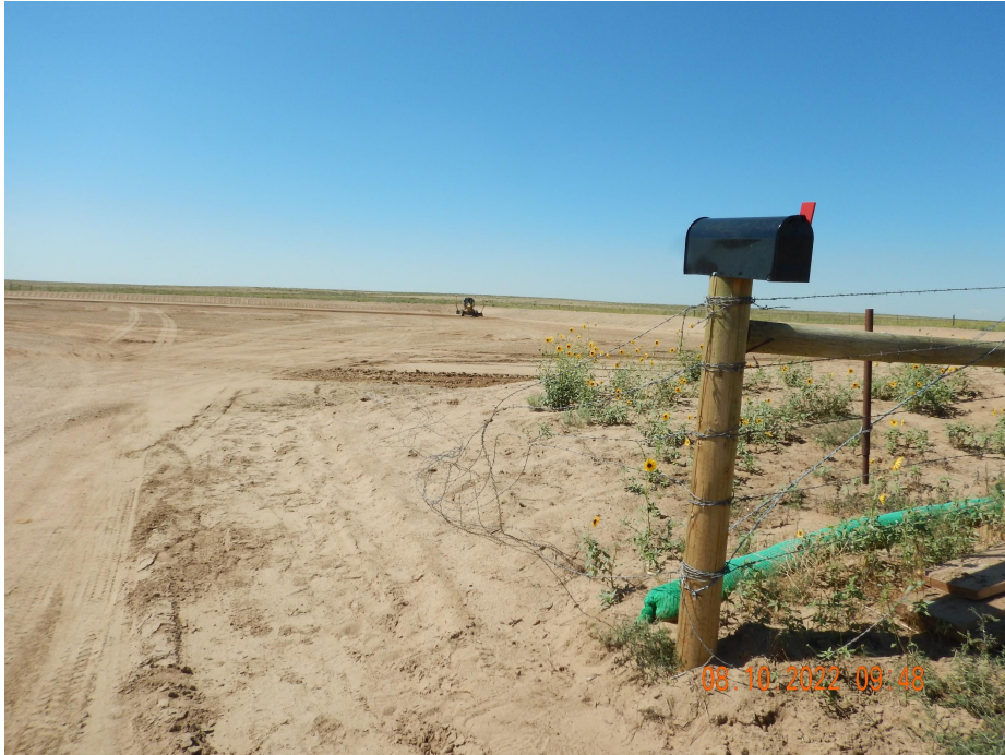
Photo 1. Photo taken from the west entrance of location, facing South. Photo illustrates Operator has installed filtrex around the entire perimeter of location and the mailbox along the entrance to comply with Rule 406.c.
