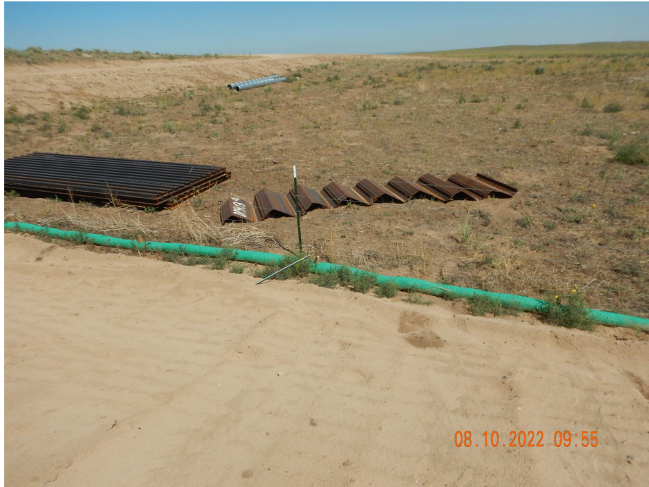
Photo 3. Photo taken from the northwestern location, facing North. Photo illustrates the cattle guard VTC to be installed and the weir stormwater BMP to be installed.
