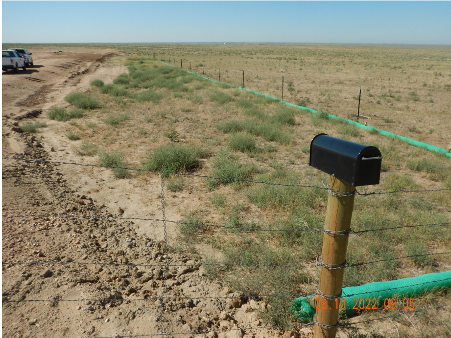
Photo 1. Photo taken from the west entrance of location, facing South. Photo illustrates Operator has installed filterrexx around the entire perimeter of location and the mailbox along the entrance to comply with Rule 406.c.
