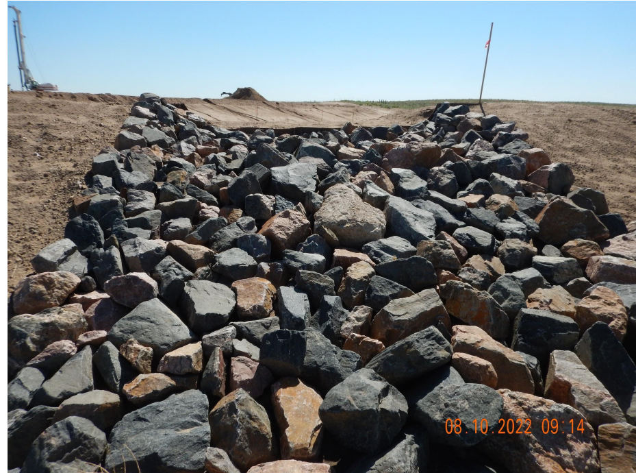
Photo 4. Photo taken from the stabilized outlet area of sediment basin.
