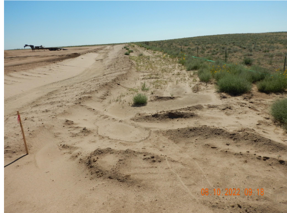
Photo 6. Photo taken from the southwestern location, facing East. See comments under Photo 5. Photo illustrates ditch maintenance is required.
