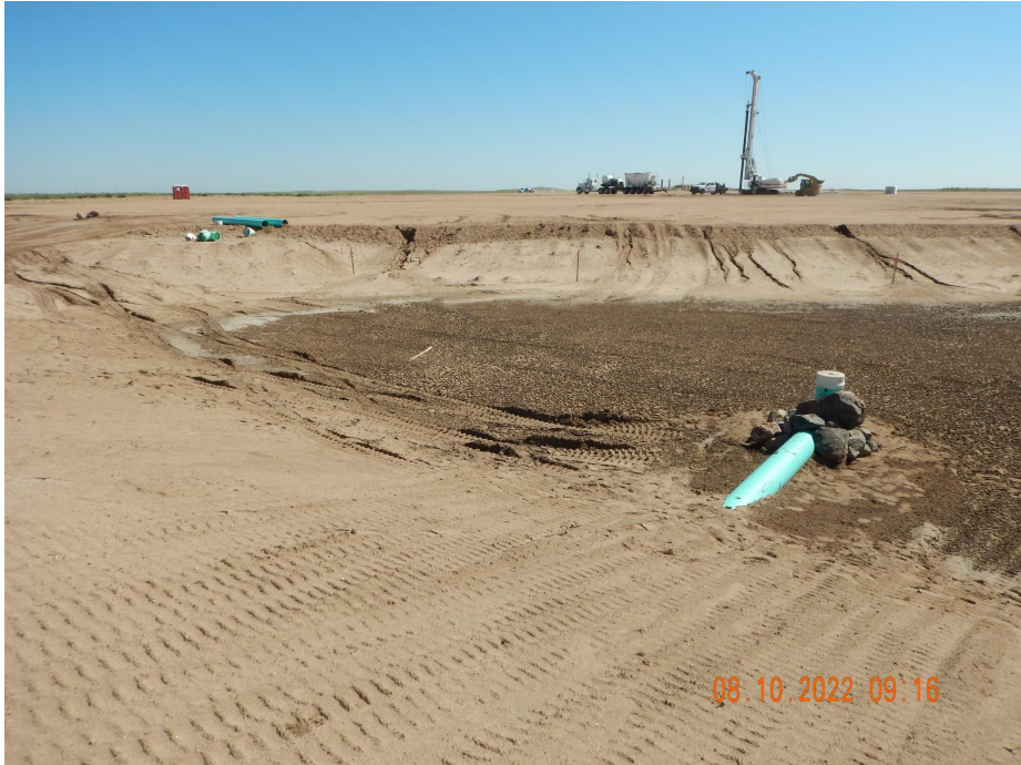
Photo 3. Photo taken from the southwestern location, facing East. Photo illustrates the sediment basin with repairs in need.
