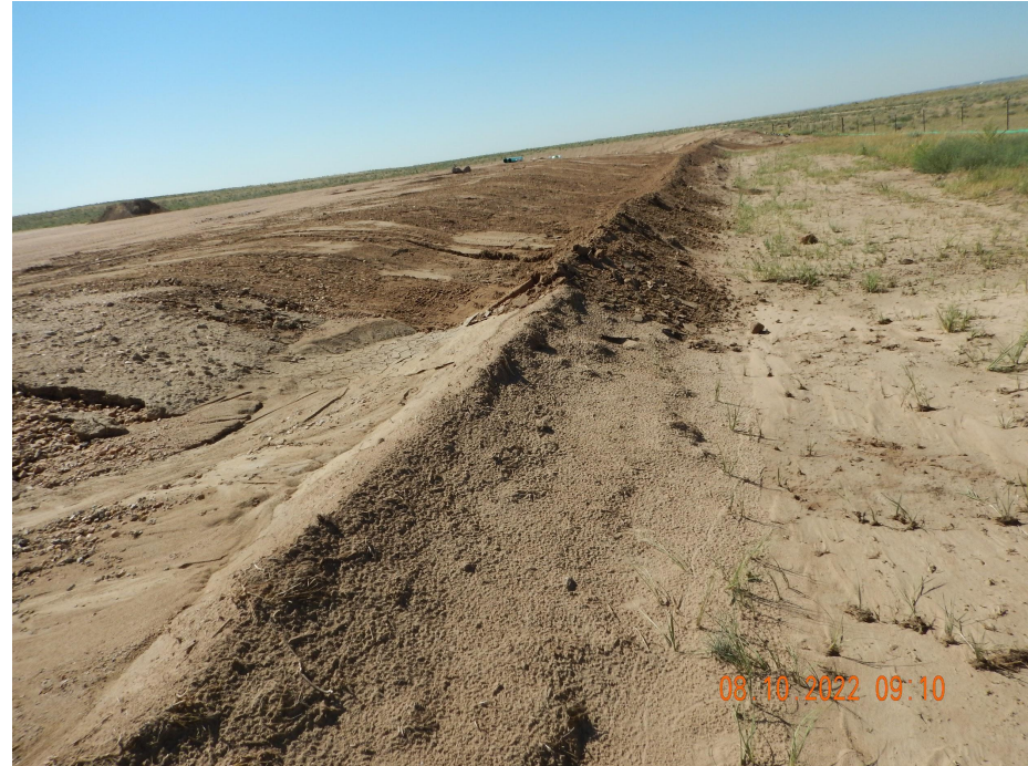
Photo 2. Photo taken from the western location, facing South. Photo illustrates Operator is in process of stormwater repairs along the fill slope and ditch BMP.
