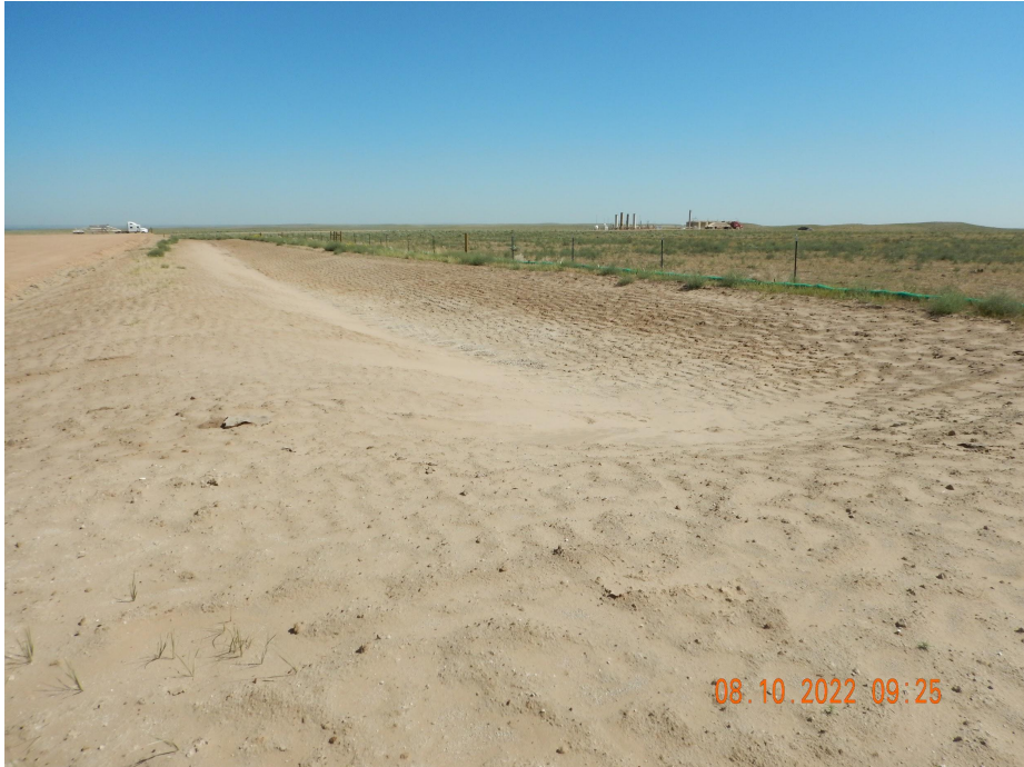
Photo 7. Photo taken from the southeastern location, facing North. Photo illustrates a run-on swale per Weld County requirements.
