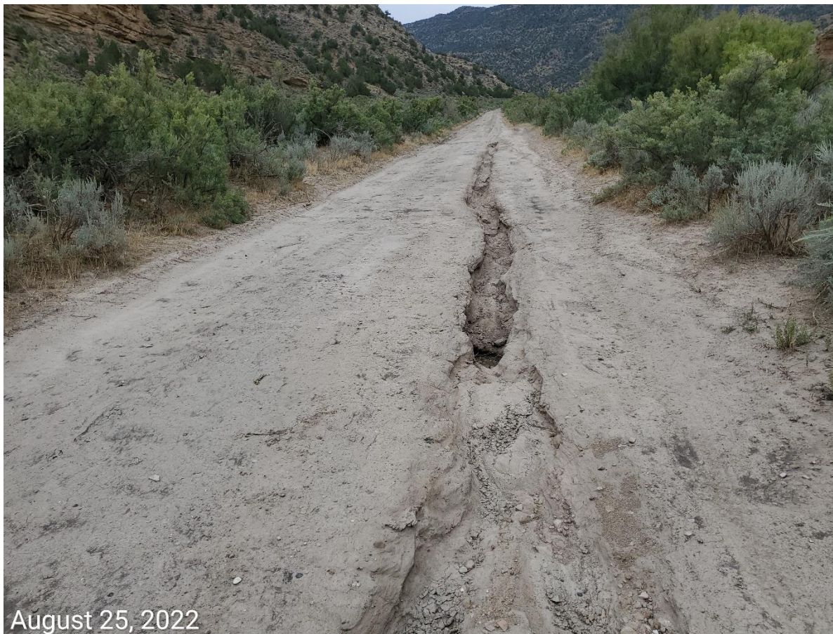
Photo 12: Photo taken from the access road south of Utah Gas Corp's Federal-Carbonera 1-2; access road is shared between the two Operators. Photo example showing erosion control and stabilization BMPs are missing or insufficient along entire access road- erosion degradation and sediment transport evident.
