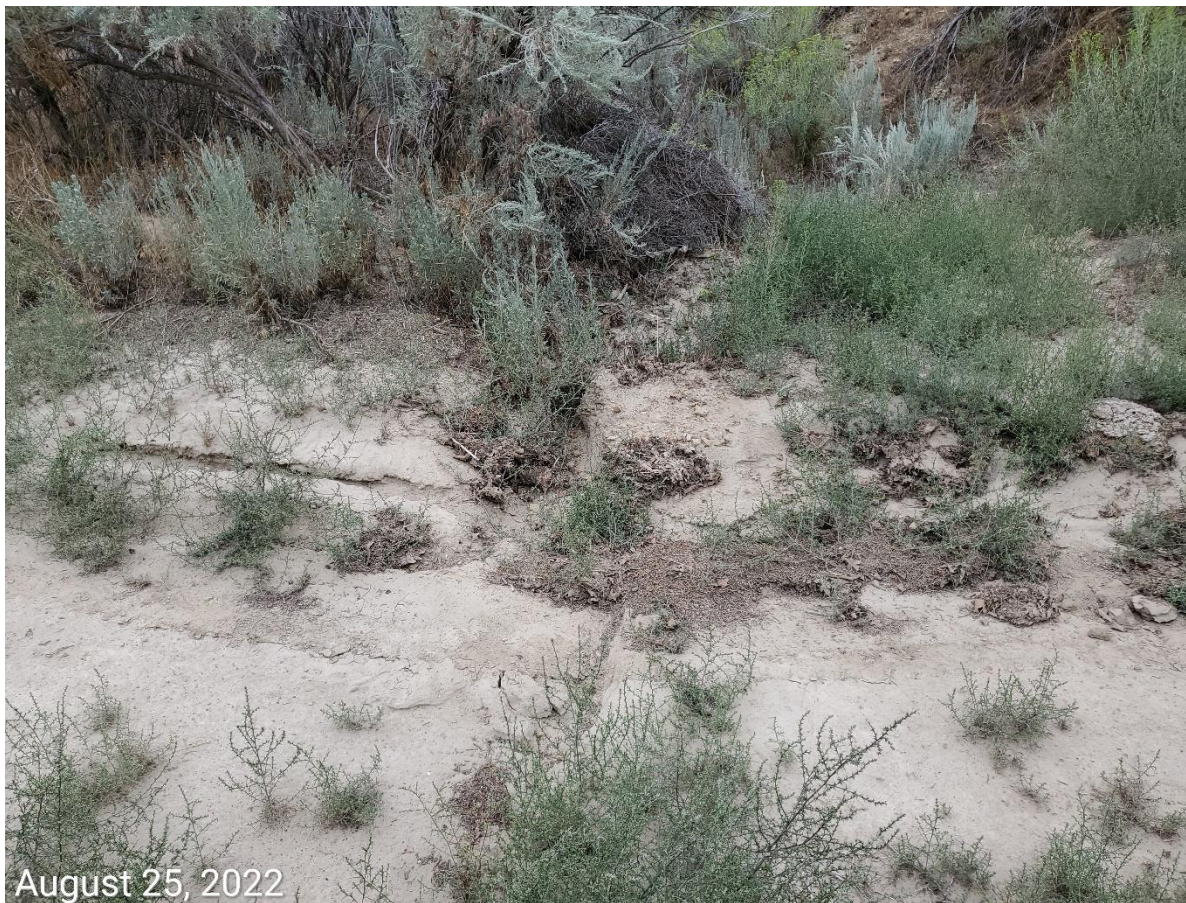
Photo 5: Photos 5-10 taken along the access road between the Government #1 and Government #2 Locations. Photos examples showing erosion control and stabilization BMPs are missing or insufficient along entire access road- erosion degradation and sediment transport evident.
