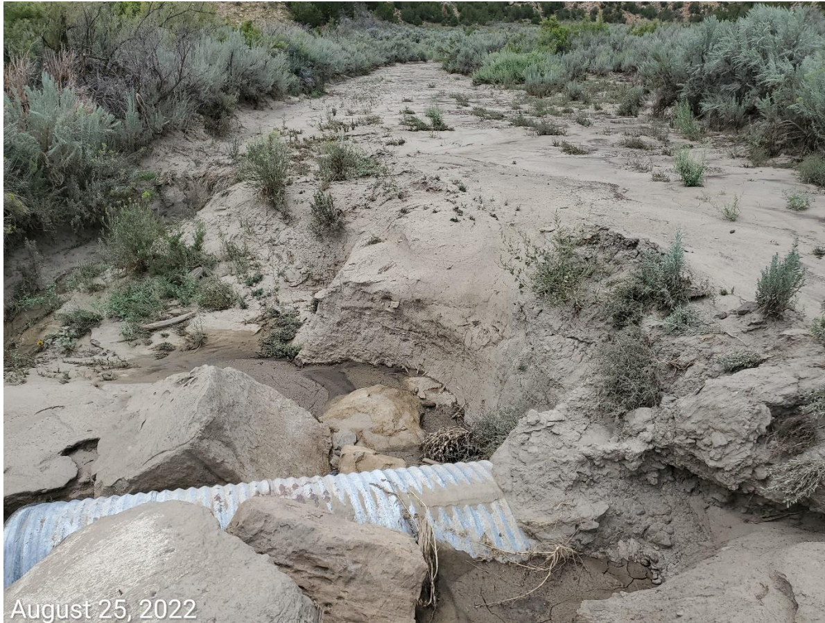
Photo 5: Stormwater erosion degradation at the access road.
