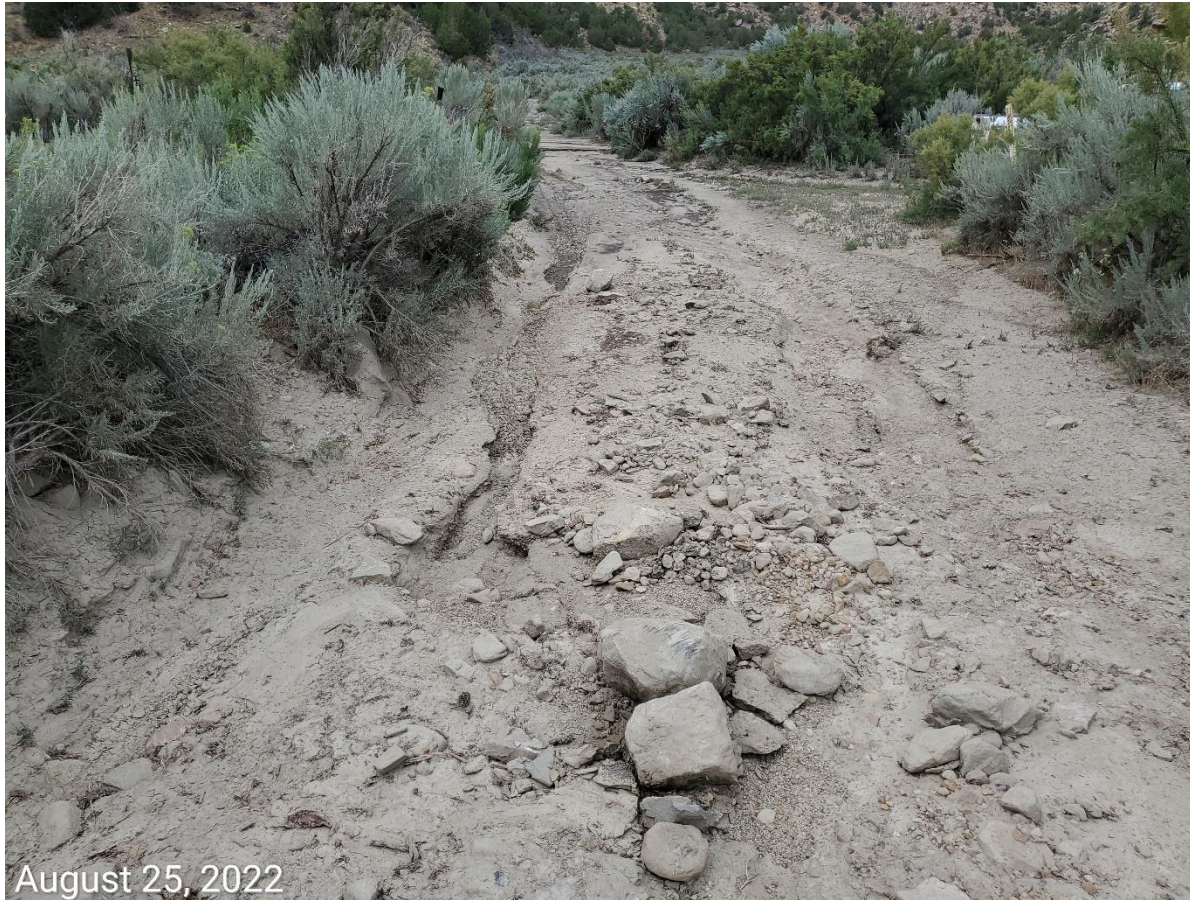
Photo 1: Stormwater erosion degradation at the access road.
