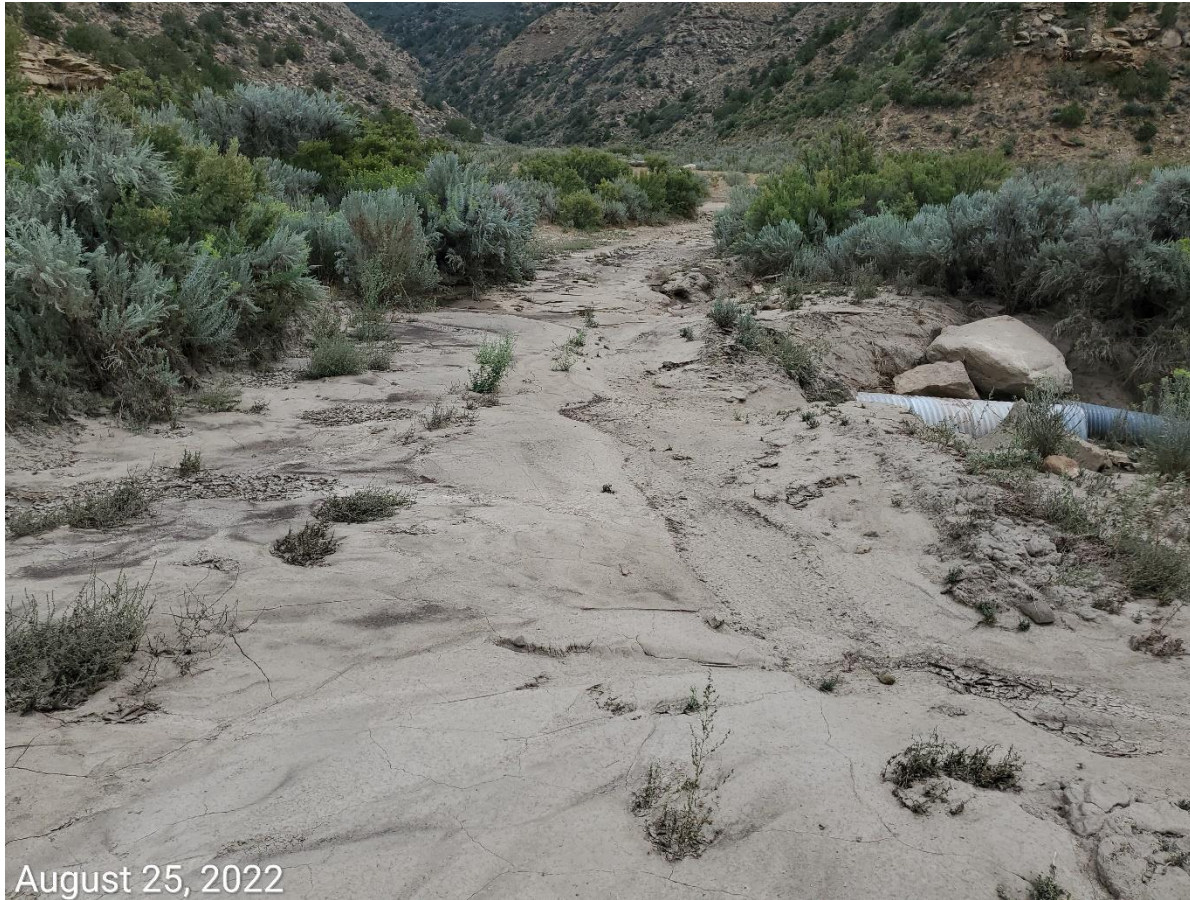
Photo 4: Stormwater erosion degradation at the access road.
