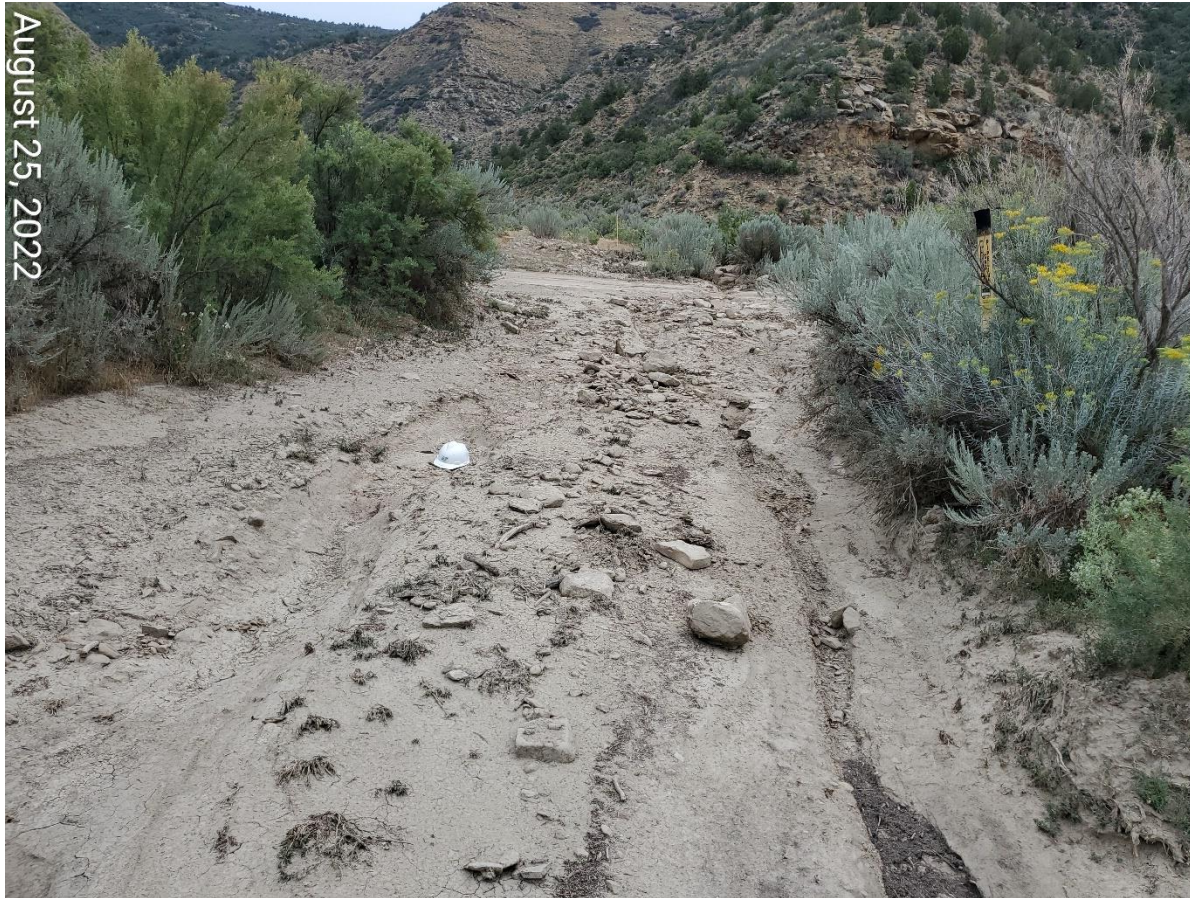
Photo 2: Stormwater erosion degradation at the access road. Hard hat in photo for scale/reference.
