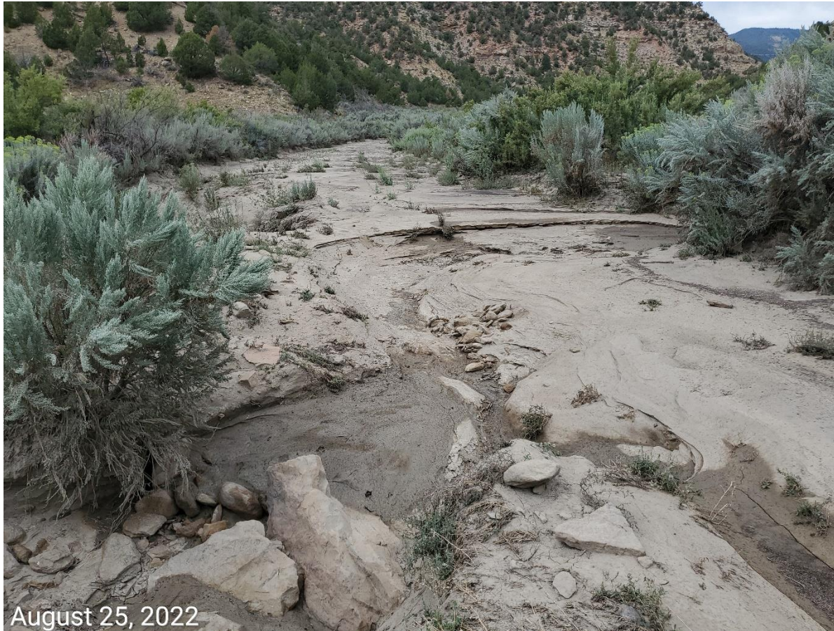
Photo 3: Stormwater erosion degradation at the access road.
