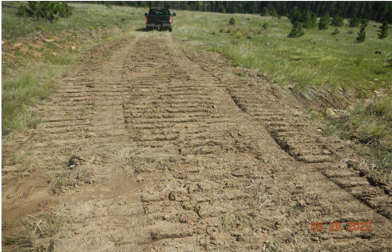
Photo 1. There has been work done to repair erosion at the water bars.
