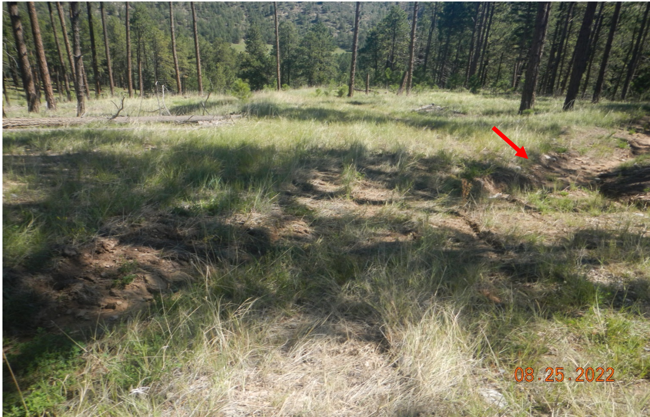
Photo 2. Additional stabilization should be performed at the red arrow where stormwater is diverted toward.
