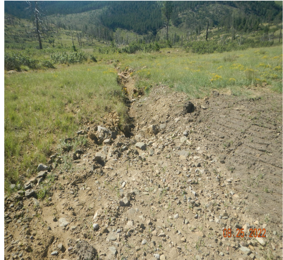
Photo 5. There is still part of the erosion channel that needs to be repaired and stabilized at the southeast portion of the location.
