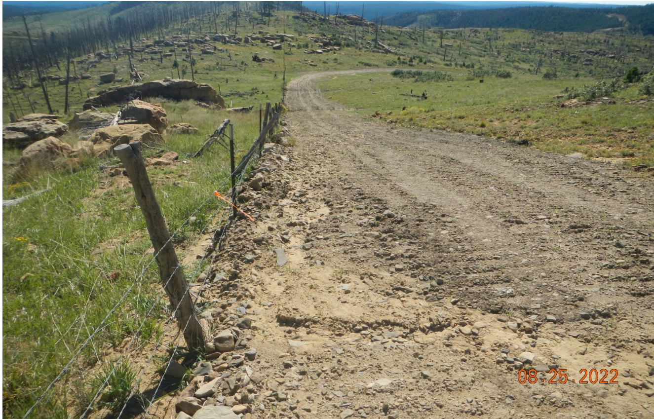
Photo 1. Facing southeast along the pre-existing access road. There are water bars installed along the road however, this area stormwater is overtopping the water bar.
