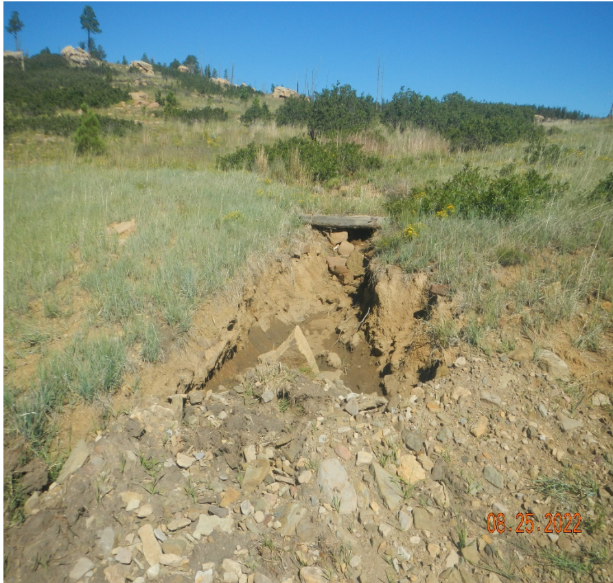
Photo 4. There is still part of the erosion channel that needs to be repaired and stabilized at the north portion of the location.
