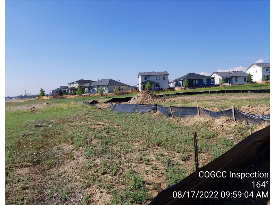
Photo 18 – Downed silt fence
