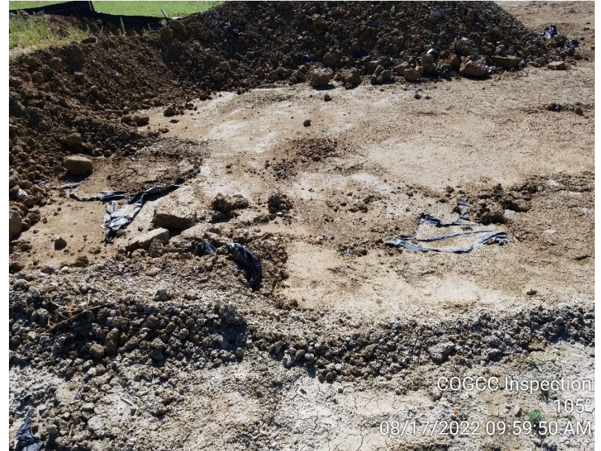
Photo 14 – Ripped lining at soil stockpile
