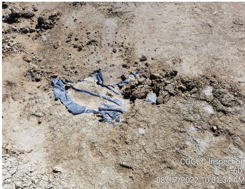
Photo 15 – Ripped lining at soil stockpile
