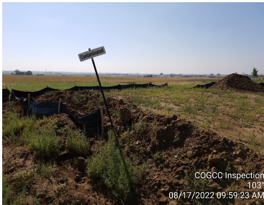
Photo 11 – Soil stockpile with 'Contaminated' sign
