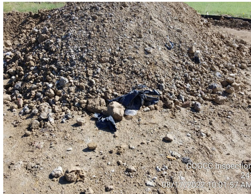
Photo 16 – Soil stockpile with ripped lining and inadequate stormwater BMPs
