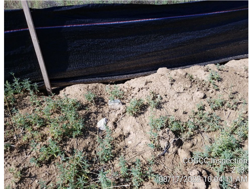
Photo 22 – Improperly installed silt fence
