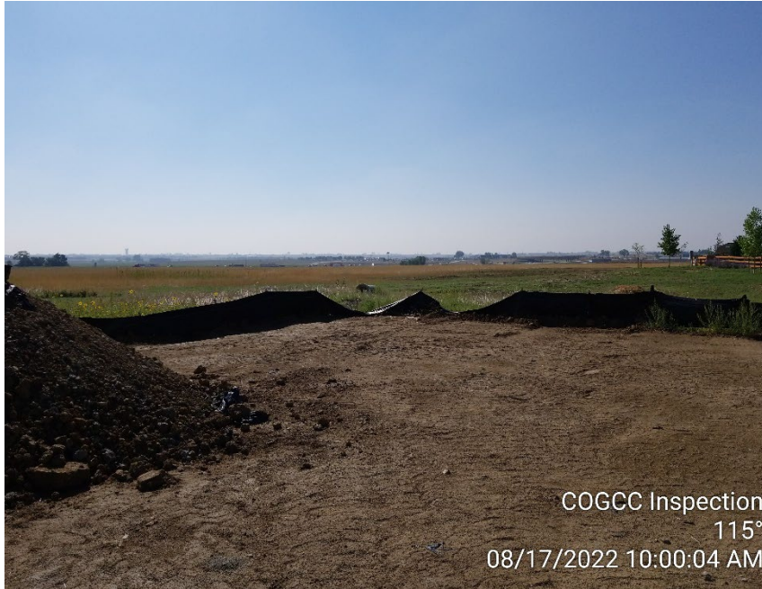
Photo 17 – Downed silt fence
