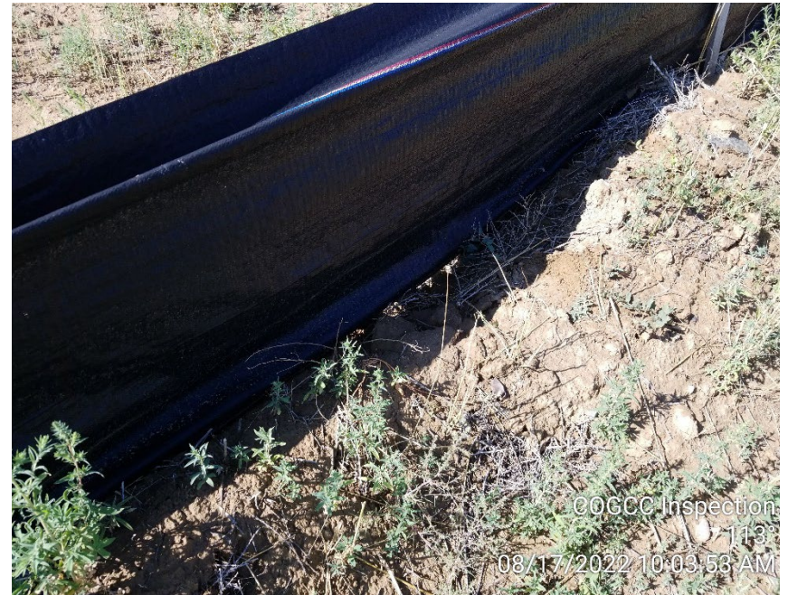
Photo 20 – Improperly installed silt fence
