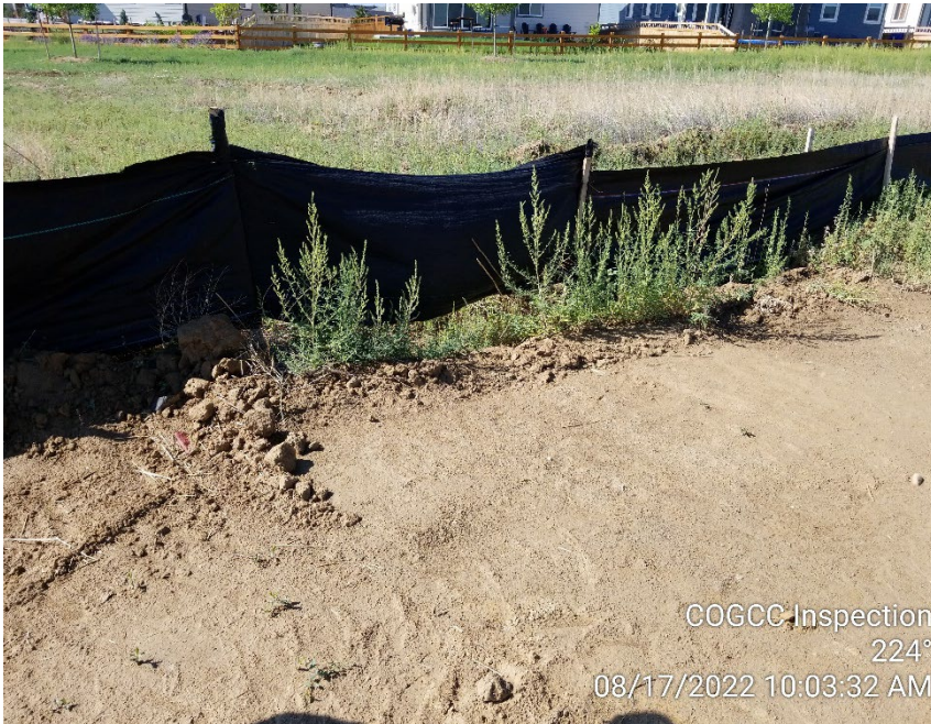
Photo 19 – Improperly installed silt fence
