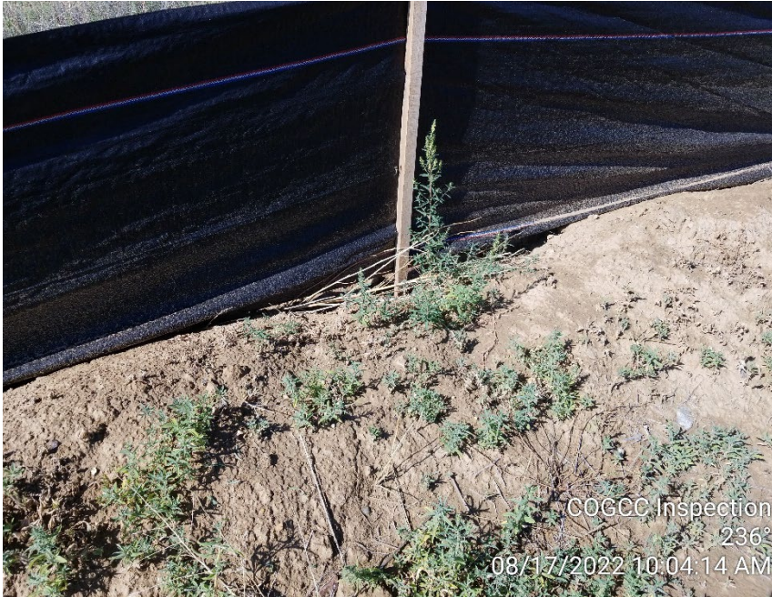
Photo 21 – Improperly installed silt fence
