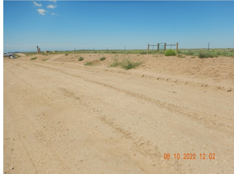
Photo 11. Photo taken from the northern location, facing West. Cut slopes are been temporarily stabilized with equipment tracking.
