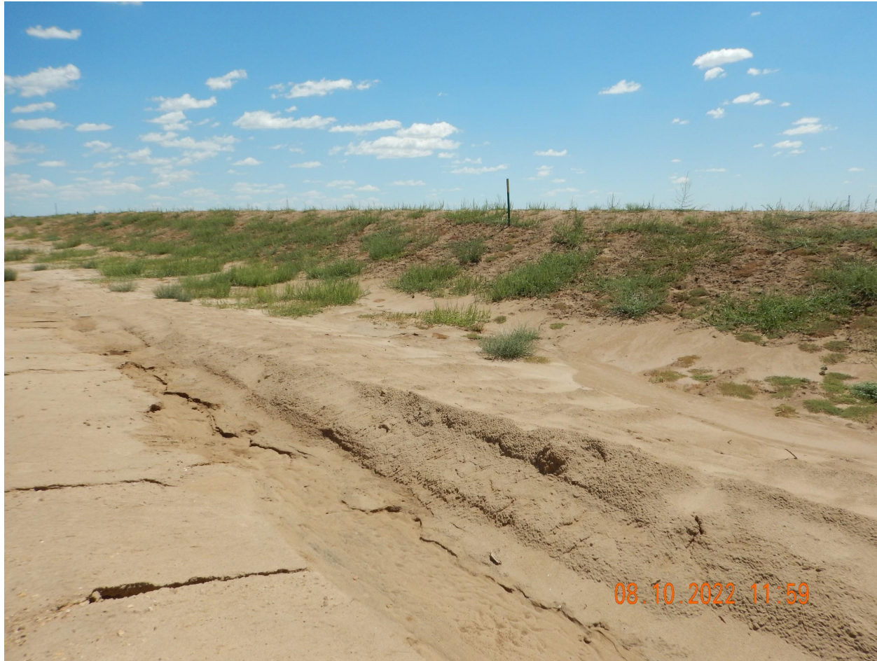
Photo 9. Photo taken from the southern location, facing Southeast. Photo illustrates that the topsoil stockpile needs to be stabilized as topsoil is starting to erode into the stormwater ditch.
