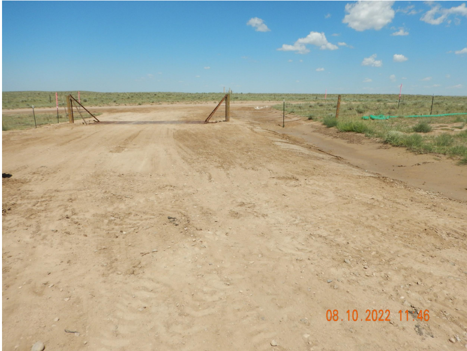
Photo 1. Photo taken from the west entrance of location, facing North. Photo illustrates a cattle guard which would also serve as a VTC device BMP.
