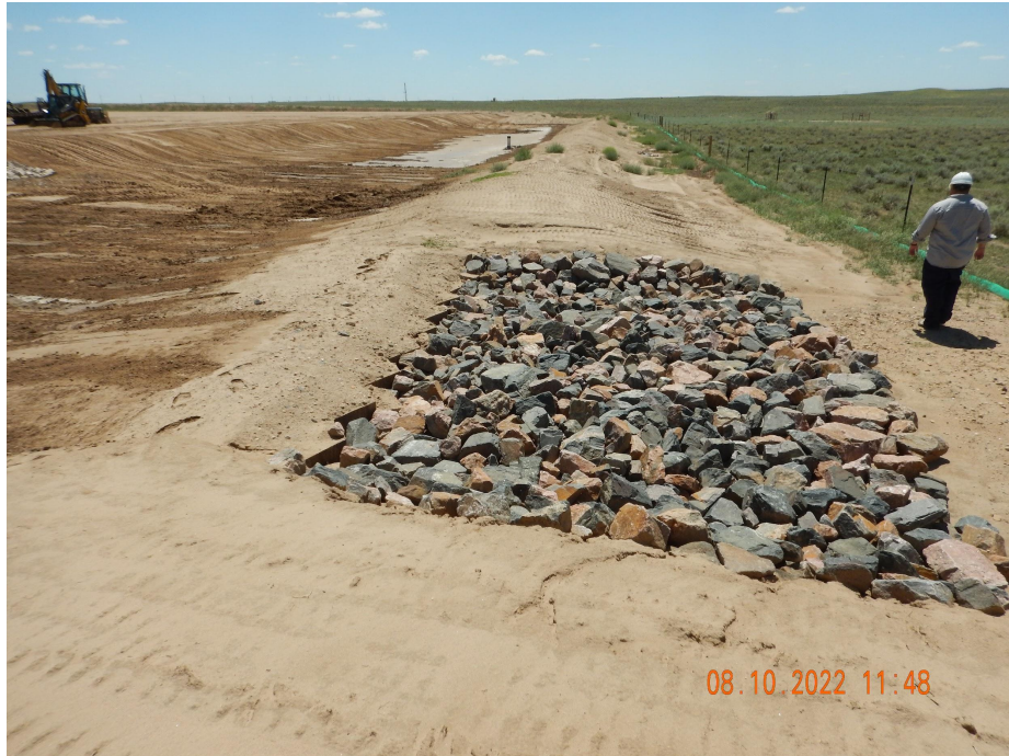
Photo 3. Photo taken from the western location, facing South. Photo illustrates the stabilized outlet of the sediment basin which appears to be in proper functioning condition.
