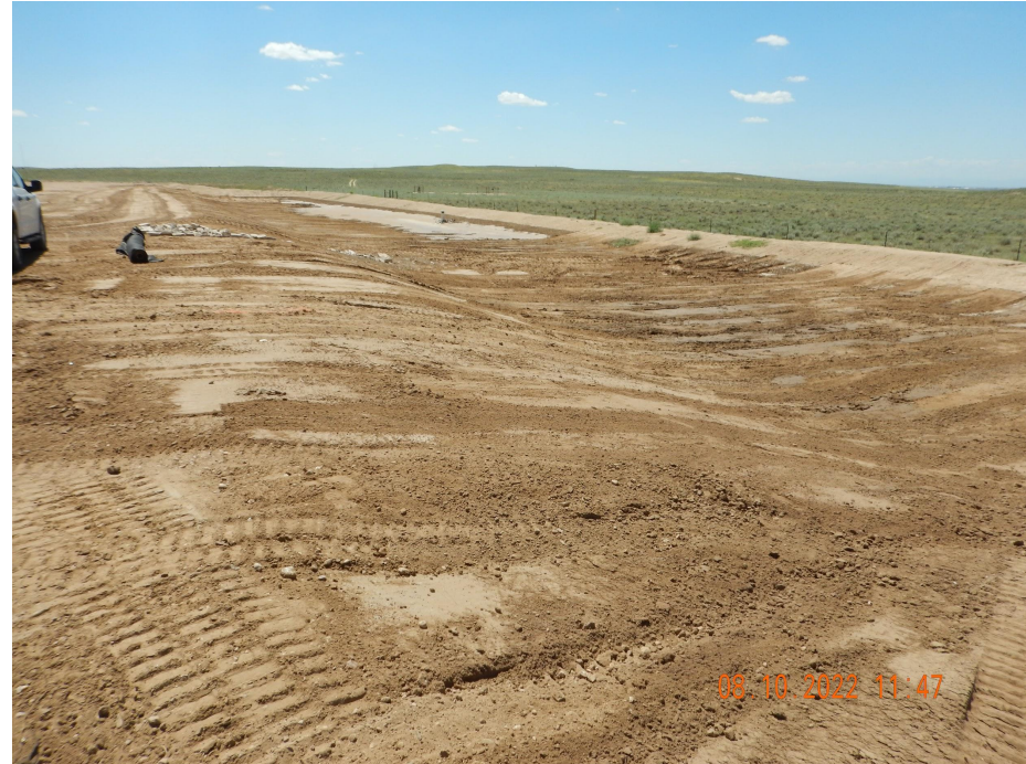
Photo 2. Photo taken from the northwestern location, facing South. Photo illustrates a sediment basin with evidence of stormwater repairs.
