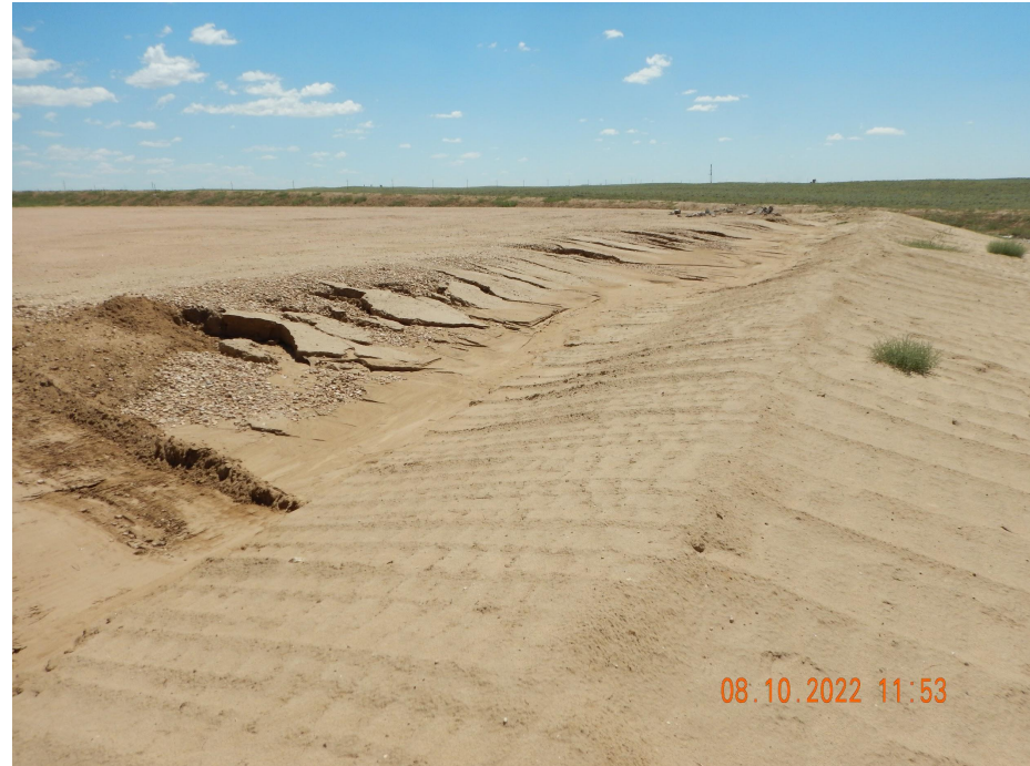
Photo 6. Photo taken from the southwestern location, facing South. Photo illustrates stormwater repairs are in process and in need of maintenance.
