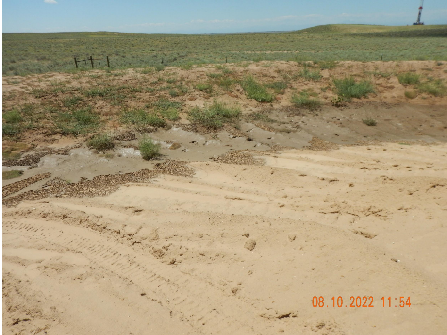
Photo 7. Photo taken from the southwestern location, facing Southwest. Photo illustrates the topsoil stockpile with weed establishment. The temporary BMP (equipment tracking) is no longer in proper functioning condition. Stockpile needs to be stabilized as topsoil is starting to erode into the stormwater ditch.
