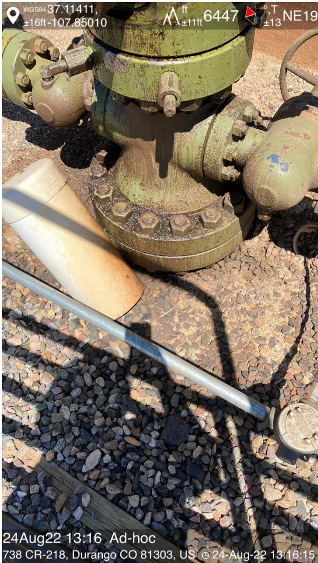
IMG 03 Lube oil
