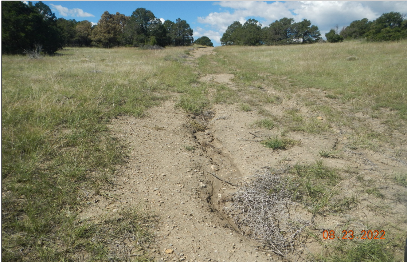
Photo 6. Facing southwest along the access road ascending toward the location. There is erosion in this area that needs to be repaired preferably without disturbing existing vegetation. The water bar further up needs maintenance.
