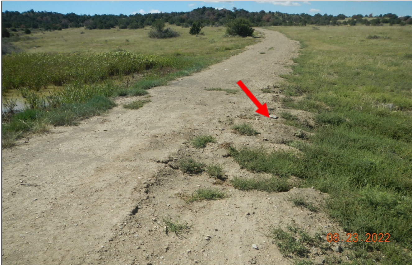
Photo 1. Facing southwest along the access road. There is erosion occurring along the road in this area at the drainage crossing. This area needs to be stabilized. Lat/Long: 37.35863, -104.53832.
