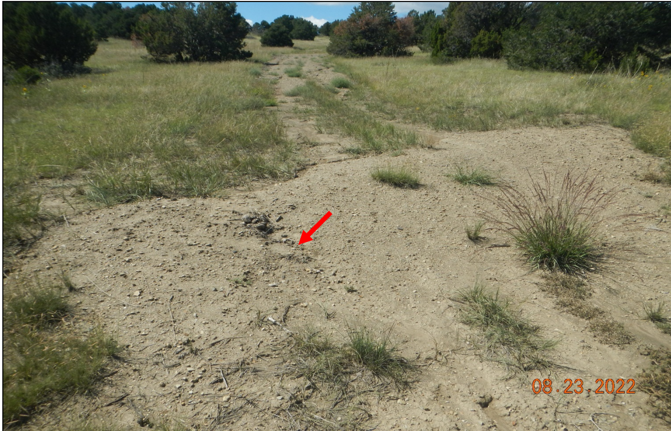
Photo 6. The water bar berm in this area needs maintenance. Stormwater is overtopping the berm causing the erosion shown in the previous photos.
