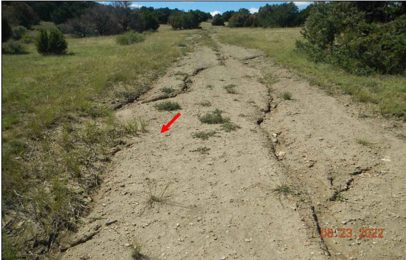
Photo 4. Facing southwest further along the access road. There is erosion occurring along the road in this area.
