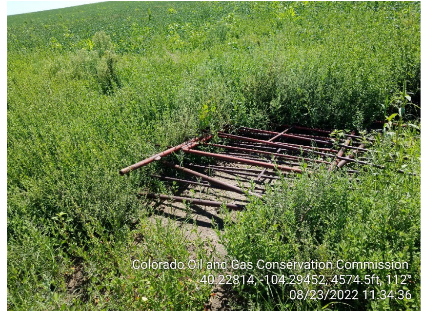
Photo 6 – Wellhead Guard off to the side covered in Weeds, Wellhead Sign no visible
