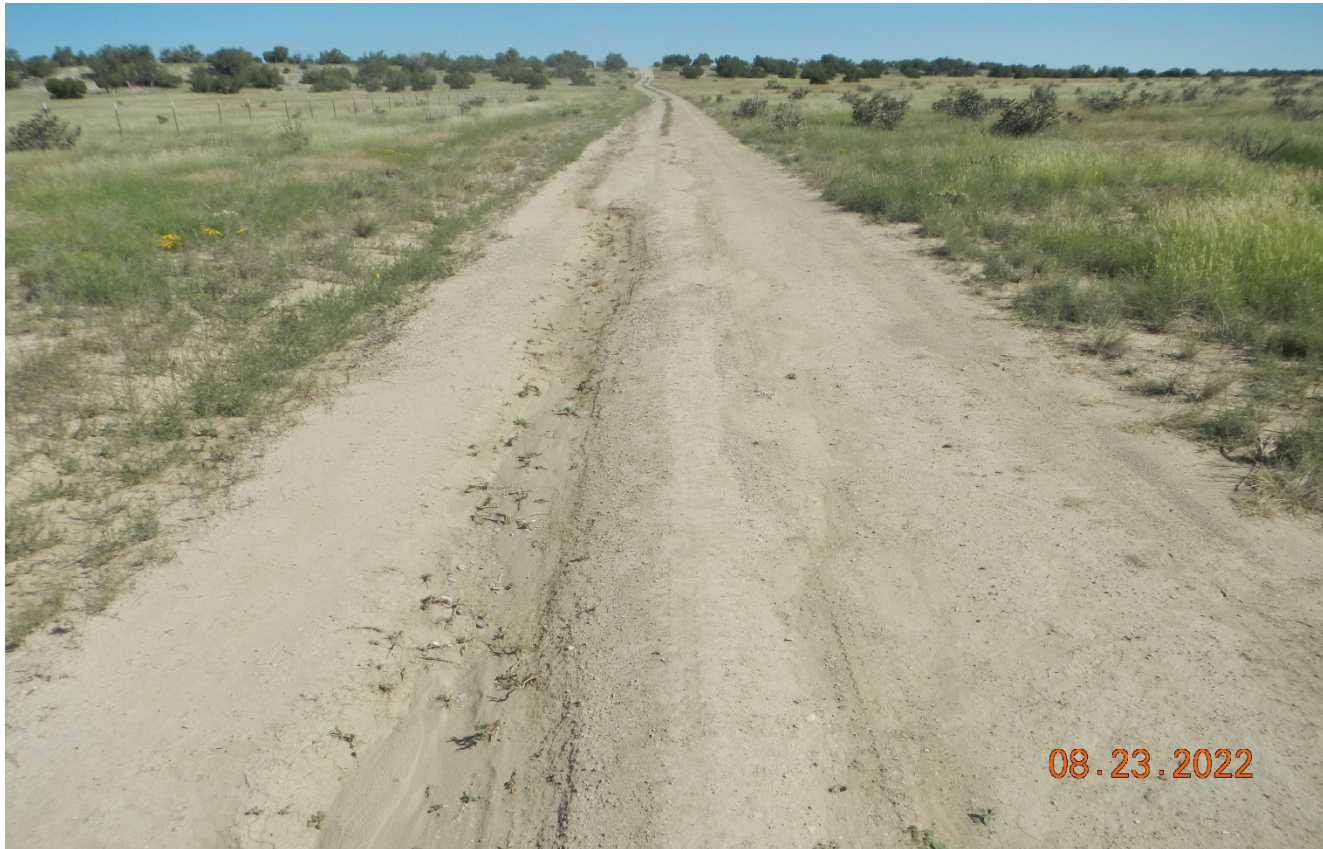
Photo 1. Facing north along the access road. There are signs of erosion along the road that need to be repaired and stabilized.
