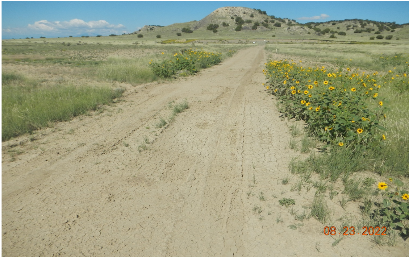
Photo 2. Facing west along the access road. There are signs stormwater is pooling along the road. The road will need to be stabilized with BMP's
