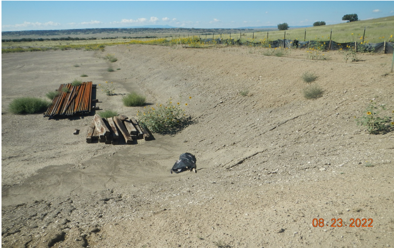
Photo 11. Northwest side of the location facing southwest toward the cut slope. The cut slope needs to be stabilized with interim reclamation. All unused equipment needs to be removed. Drill pipe, wood ties, ect.
