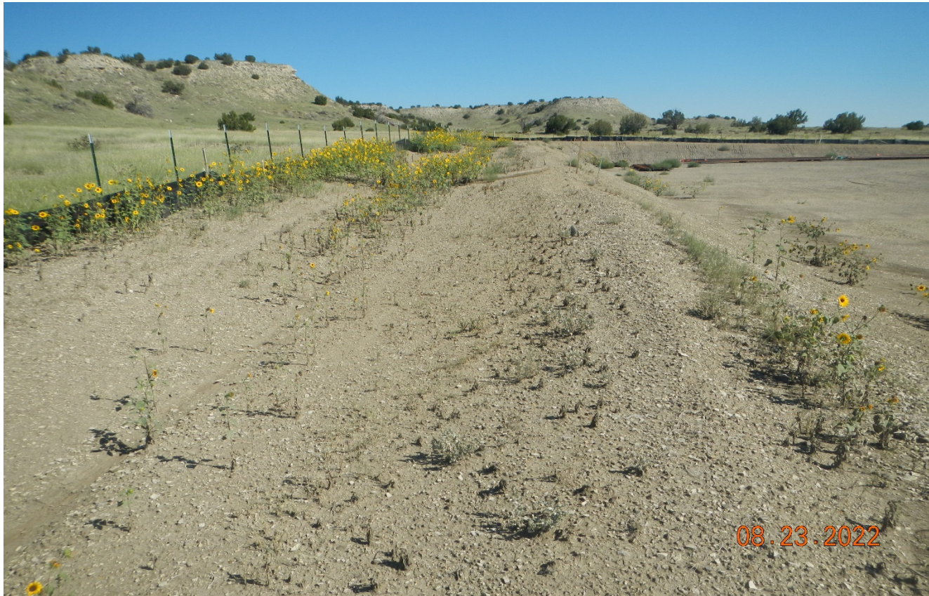
Photo 10. Southwest side of the location facing northwest. There are wattles installed along the perimeter swale. The disturbed soils will need to be reclaimed for long term stabilization.
