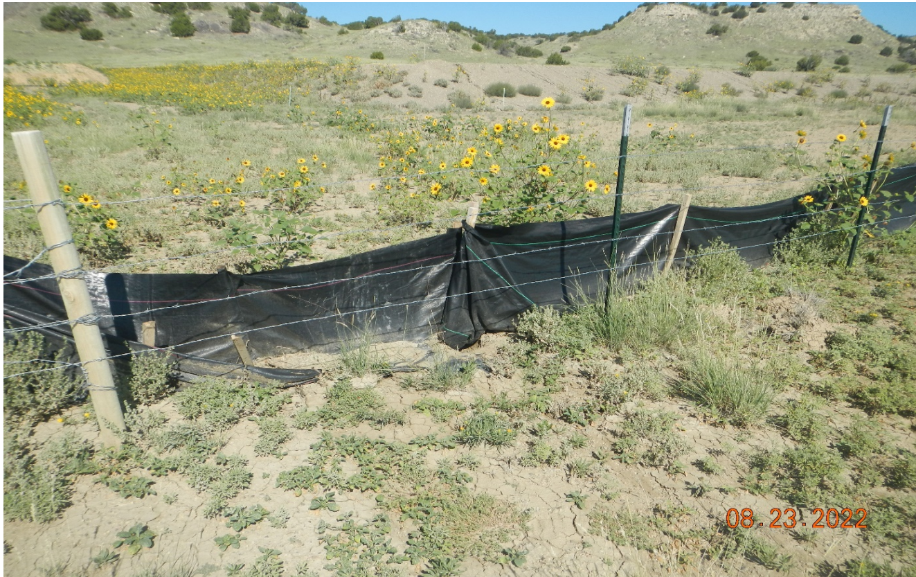
Photo 5. Facing northwest at the southeast corner of the location. Stormwater is being concentrated to this area. The silt fence is not adequate and additional BMP's need to be installed in this area.
