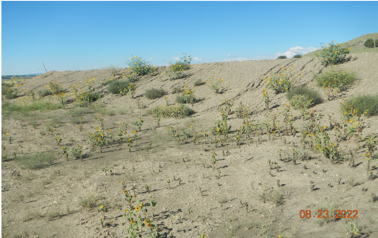
Photo 4. Facing southwest toward the fill slope of the well pad. There is erosion occurring along the fill slope. The fill slope needs to be recontoured and stabilized for interim reclamation.
