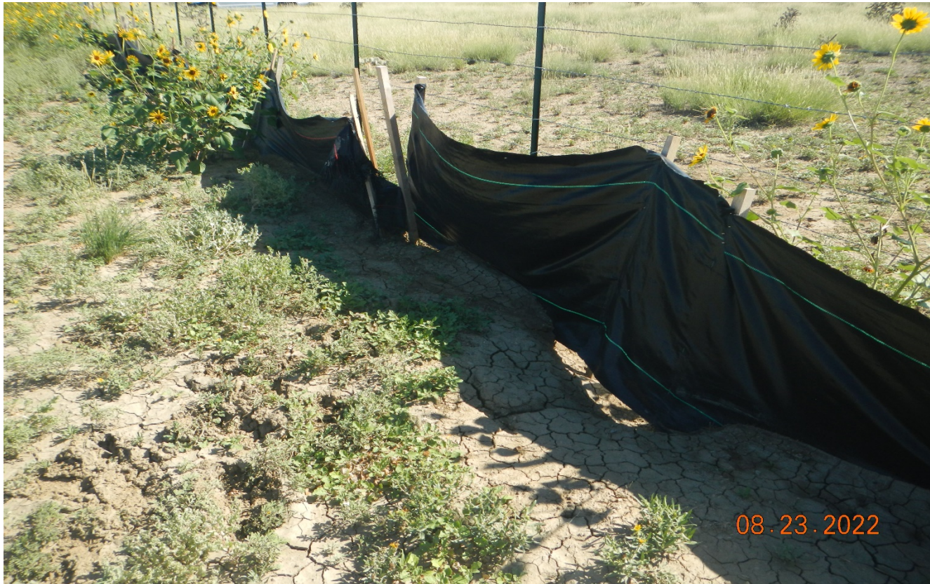
Photo 6. Stormwater is flowing underneath the silt fence in the southeast corner of the location. The silt fence is not adequate and additional BMP's need to be installed in this area. Silt fence is only a temporary erosion control and long term erosion controls need to be installed e.g. sediment trap, rock rip/rap, seeding, vegetation, ect.
