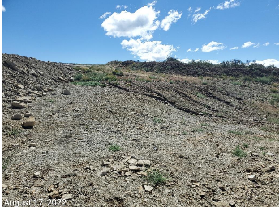
Photo 15: Photos taken from the sediment trap/basin on the south end of the Location. Photo shows inlet to the sediment trap/basin has not been properly engineered/stabilized, resulting in degradation to the control and sediment transport.
