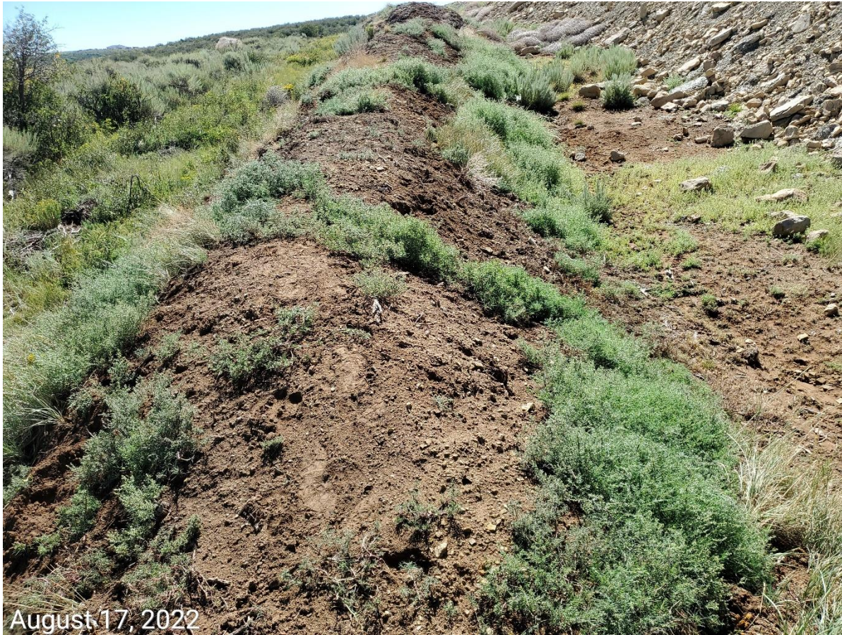
Photo 2: Photo example showing the topsoil stockpile in use as part of the perimeter stormwater ditch/berm; photo also shows weed establishment on the topsoil; BMPs to protect topsoil remain missing or insufficient.
