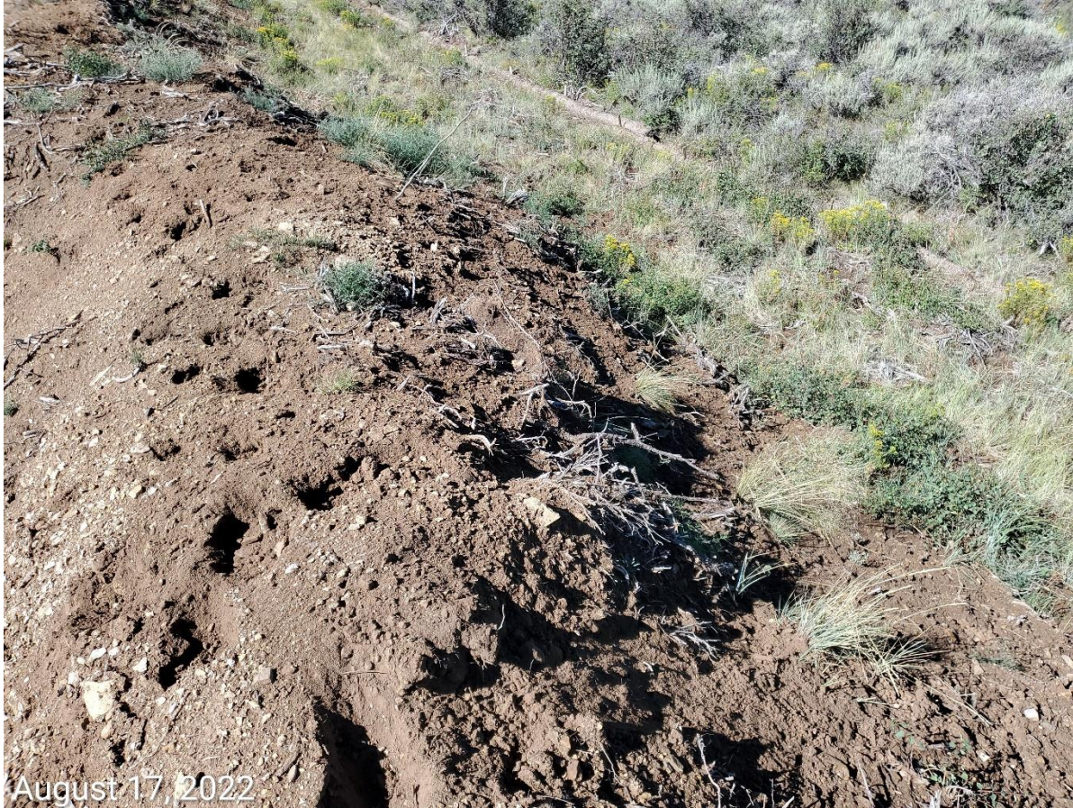
Photo 9: Photo example showing topsoil stockpiles along perimeter of the Location remain bare and exposed; BMPs to protect topsoil remains missing or insufficient; erosion degradation evident.
