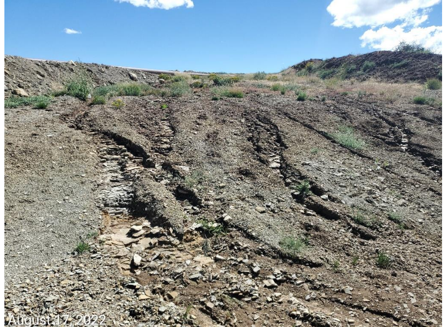
Photo 15: Photos taken from the sediment trap/basin on the south end of the Location. Photo shows inlet to the sediment trap/basin has not been properly engineered/stabilized, resulting in degradation to the control and sediment transport.
