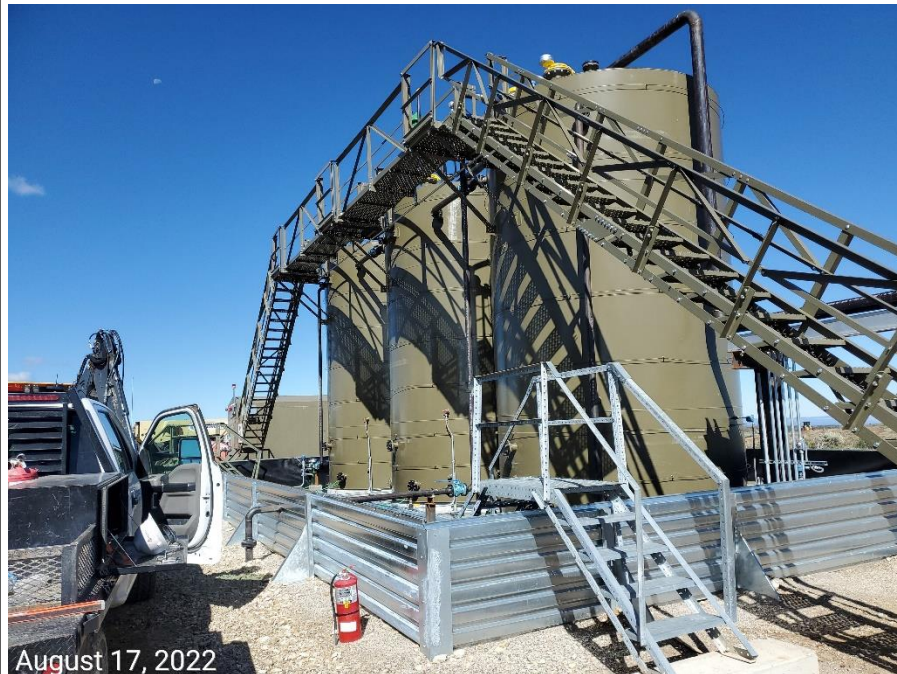
Photo 1: Tanks/Battery on the north end of the Location; tanks missing required labeling.
