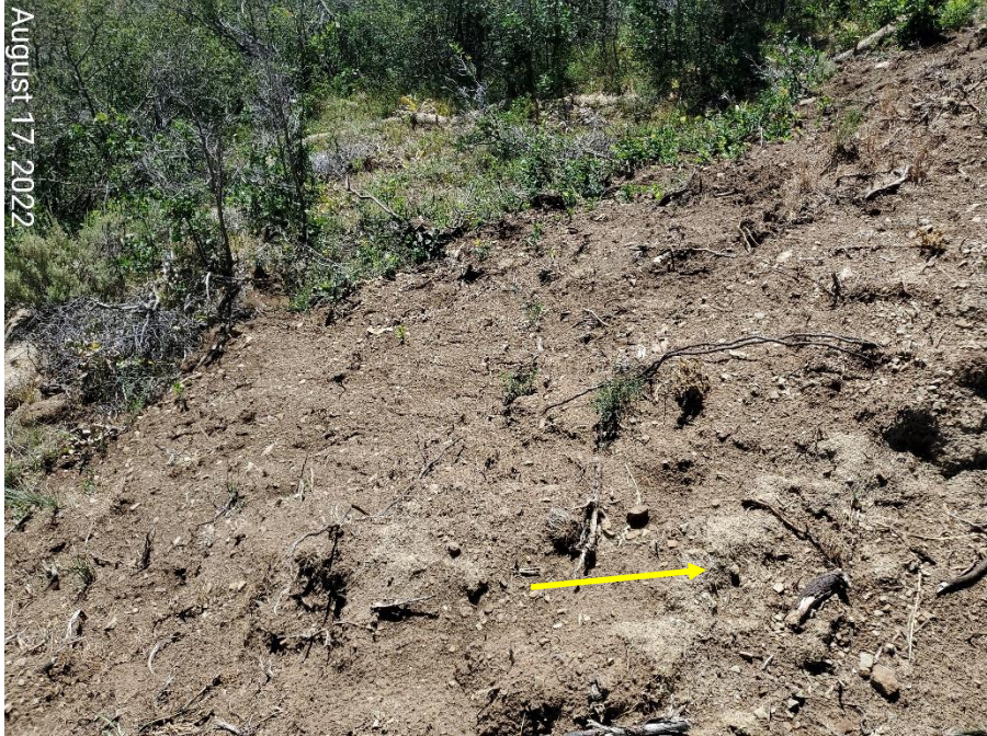
Photo 3: Photos examples showing BMPs to protect the topsoil stockpiles are missing or insufficient; soils at the stockpiles are exposed and at risk to wind and water erosion. Arrow shows areas of hydromulch that had been previously applied; BMP has not been maintained.
