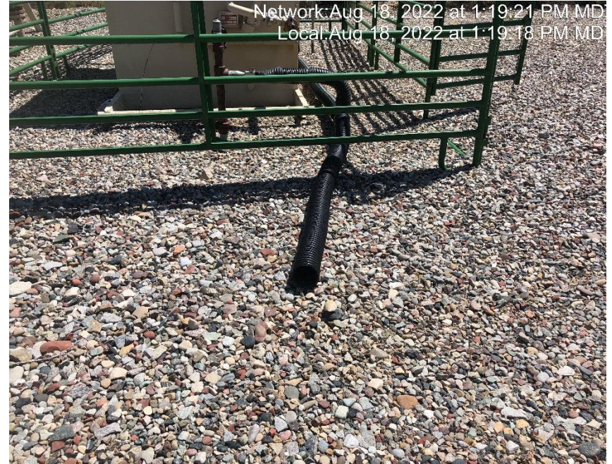
Photo #7492 Flow line heating insulation open ended and not capped.
