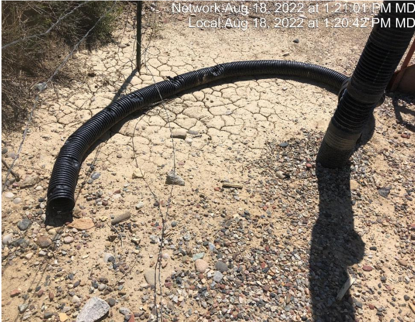
Photo #7493 Flow line heating insulation open ended and not capped.
