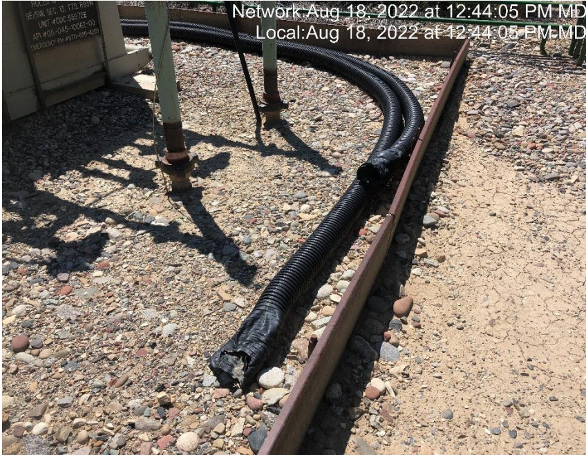
Photo #7485 Heating insulation open ended and not capped.
