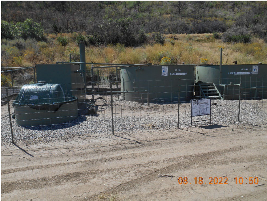
Separator and Produce water tanks
