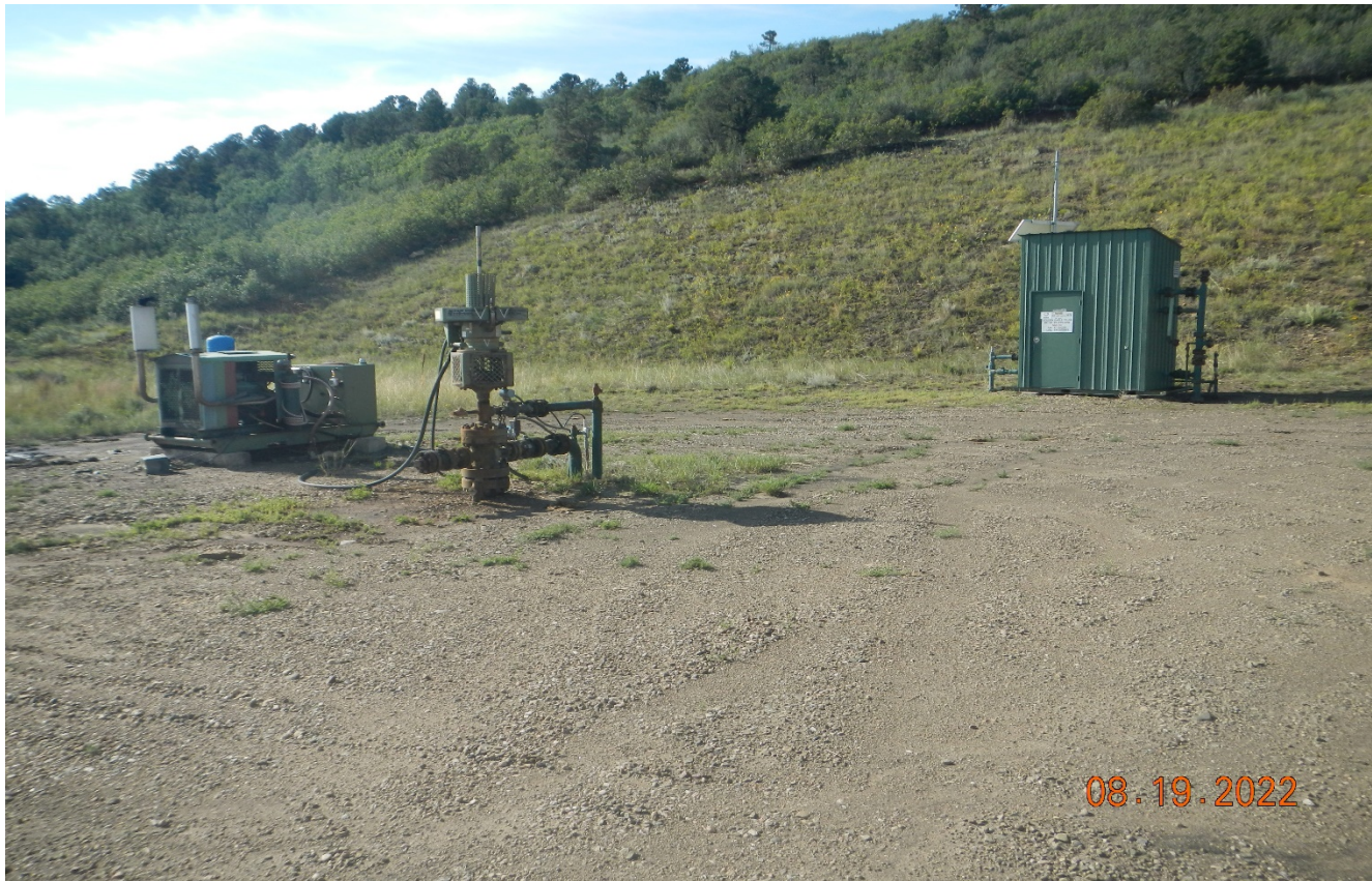
Photo 3. Facing southeast toward the wellsite.
