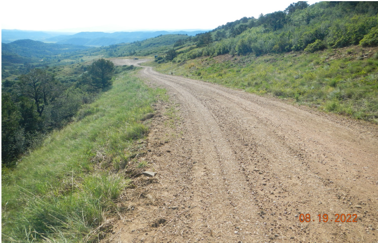
Photo 1. Facing east along the access road.
