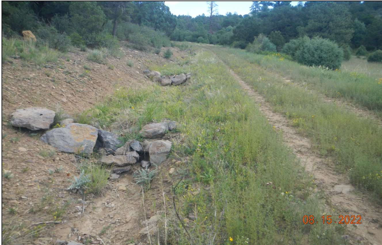
Photo 10. Facing northeast further along the access road. There is vegetation establishing along the road side and rock check dams are installed.
