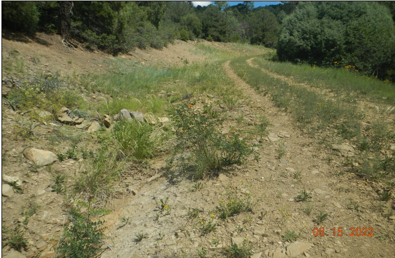
Photo 11. Facing northeast further along the access road. There is vegetation establishing along the road side and rock check dams are installed.
