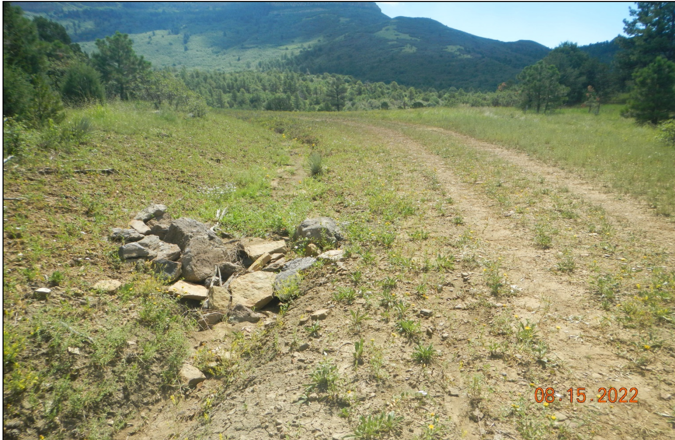
Photo 12. Facing northeast further along the access road. There is vegetation establishing along the road side and rock check dams are installed.
