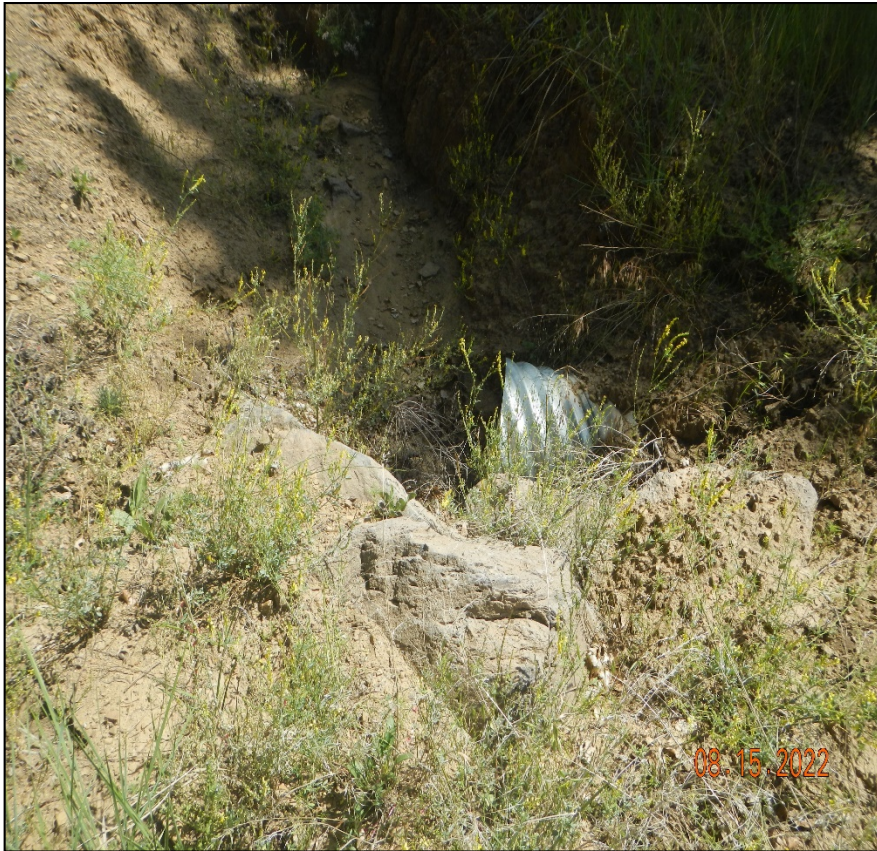
Photo 6. The culvert inlets are maintained and clear of debris and sediment.
