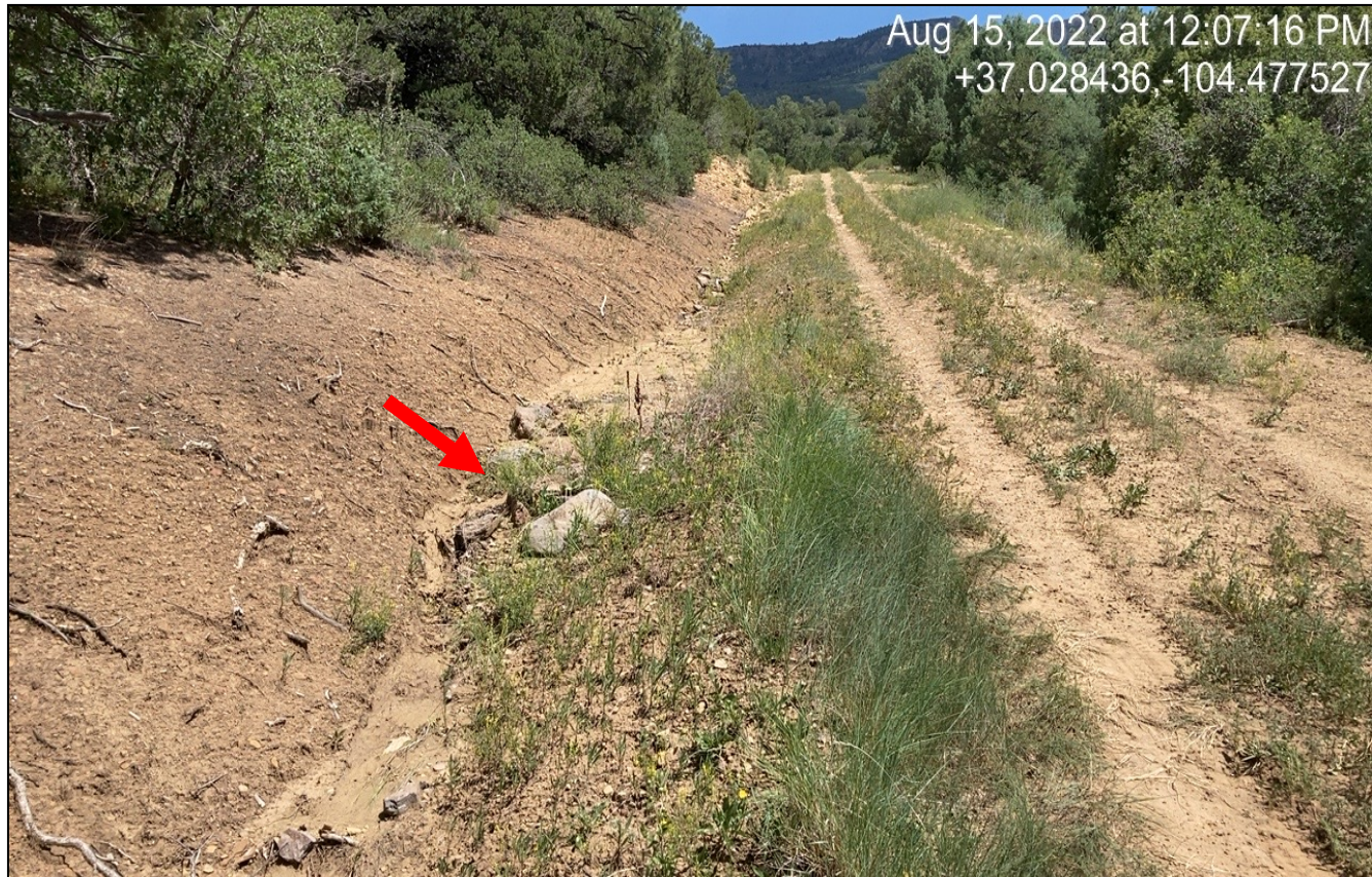
Photo 9. Facing northeast further along the access road. Some of the rock check dams are in need of maintenance. The road side along this area has not established vegetation.
