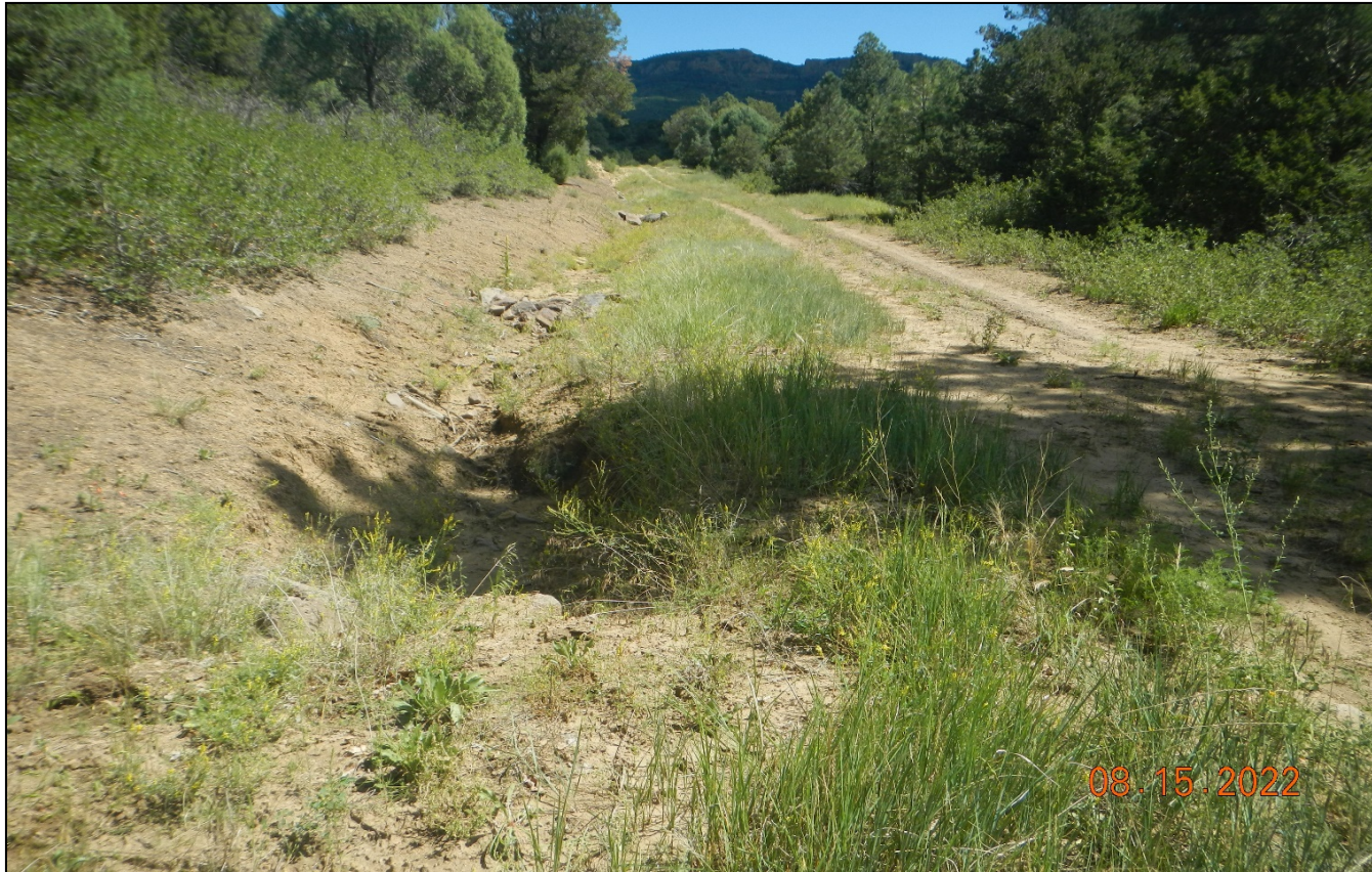
Photo 8. Facing northeast further along the access road. There is vegetation establishing along the road side and rock check dams are installed.
