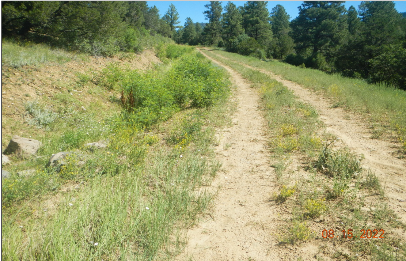
Photo 4. Facing northeast further along the access road. There is vegetation establishing along the road side and rock check dams are installed.
