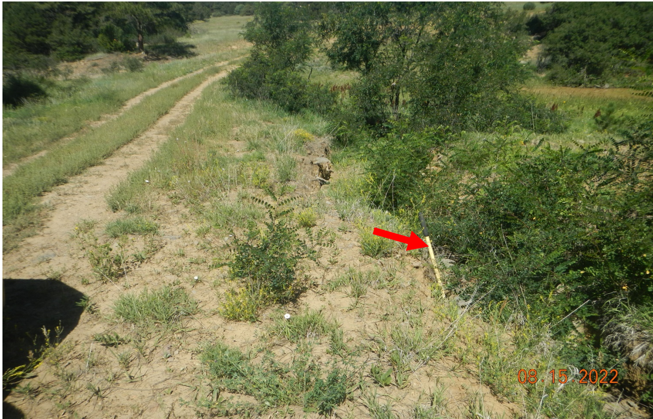
Photo 1. There is an erosional gully along the access road that was not repaired at Lat/Long:37.02219,-104.48216. Arrow points to 4.5 ft shovel.
