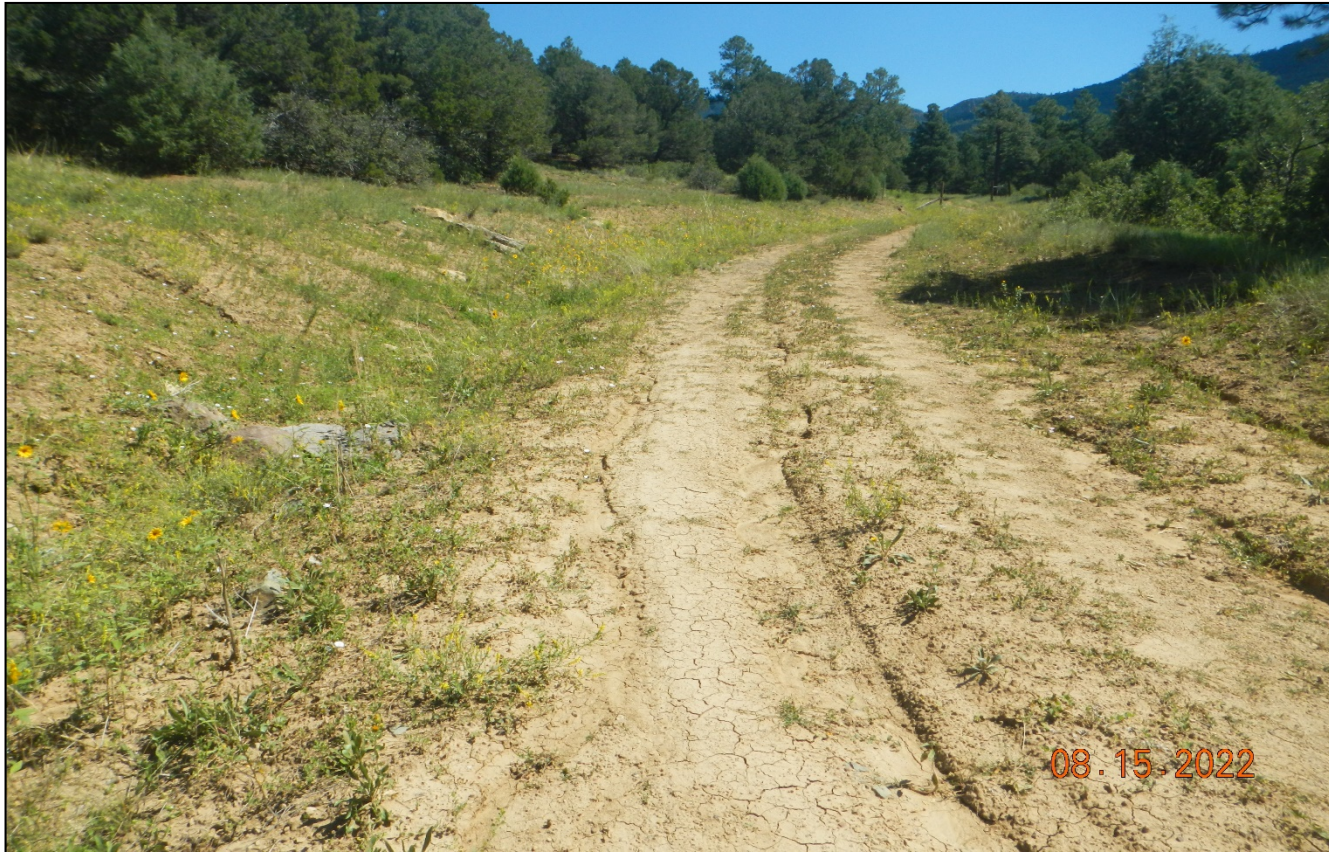
Photo 3. Facing northeast along the access road. There is vegetation establishing along the road side and rock check dams are installed.
