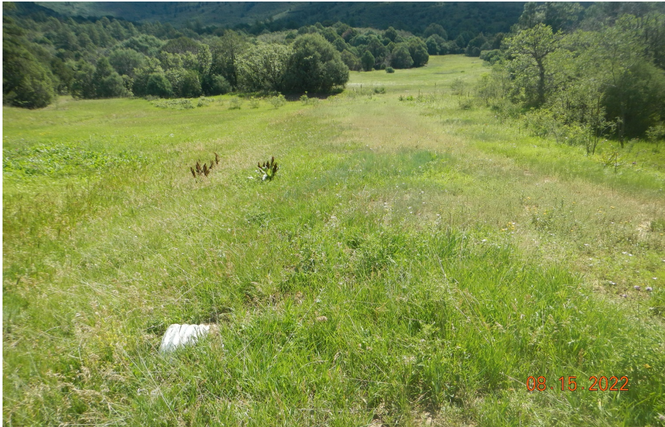
Photo 1. Facing east along the former access road. The pre-existing road is stabilized with perennial vegetation. A culvert is installed at the drainage crossing.
