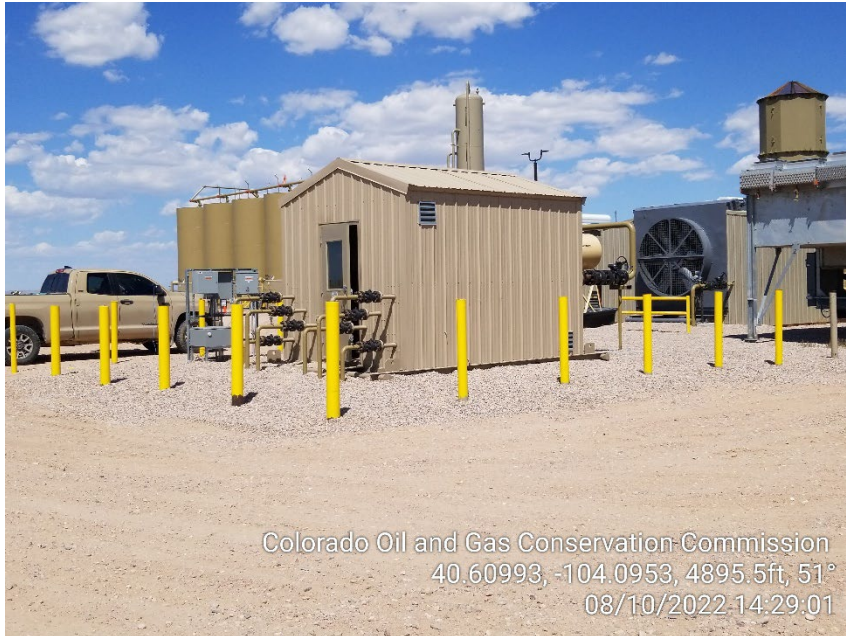
Photo 7 – Gas Lift Injection Meter House
