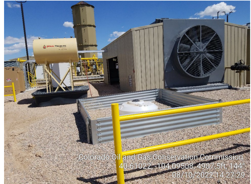
Photo 4 – Drain Pit – Missing Labels
