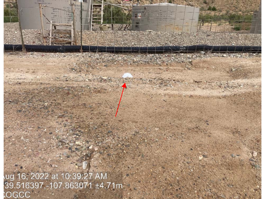
Subsidence at tanks (hard hat in subsidence)
