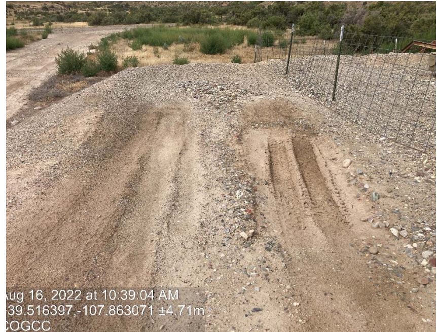
Subsidence at tanks
