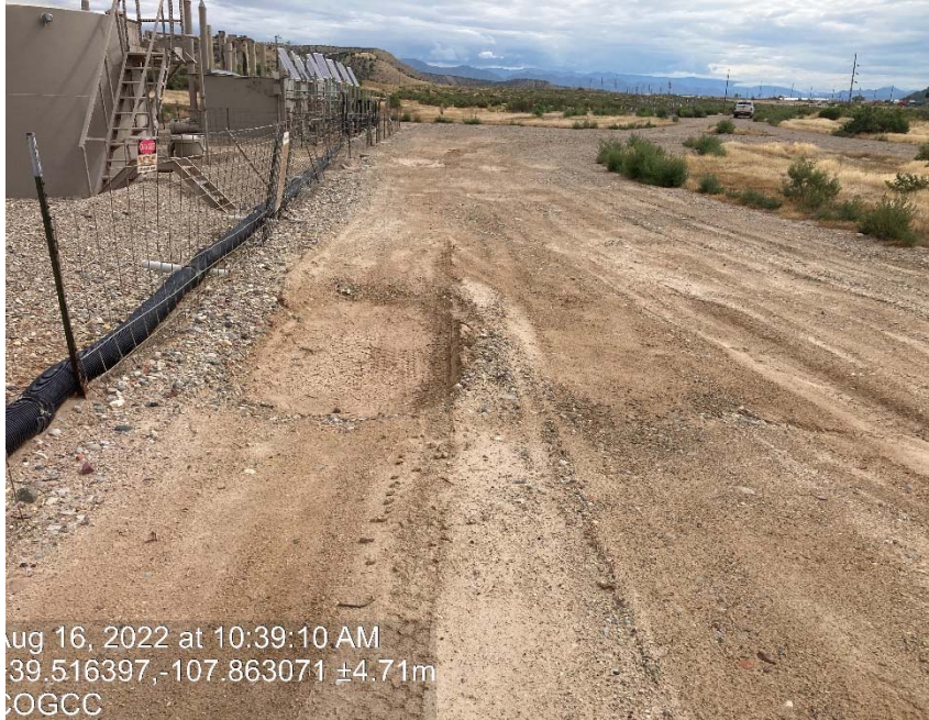
Subsidence at tanks
