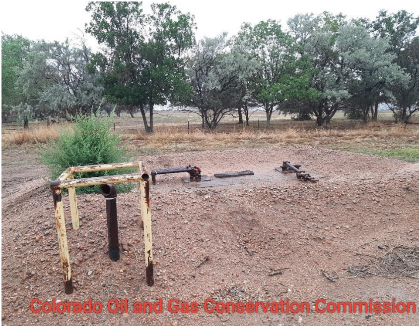
Photo 5 Cement vault not placards or tank volume markings
