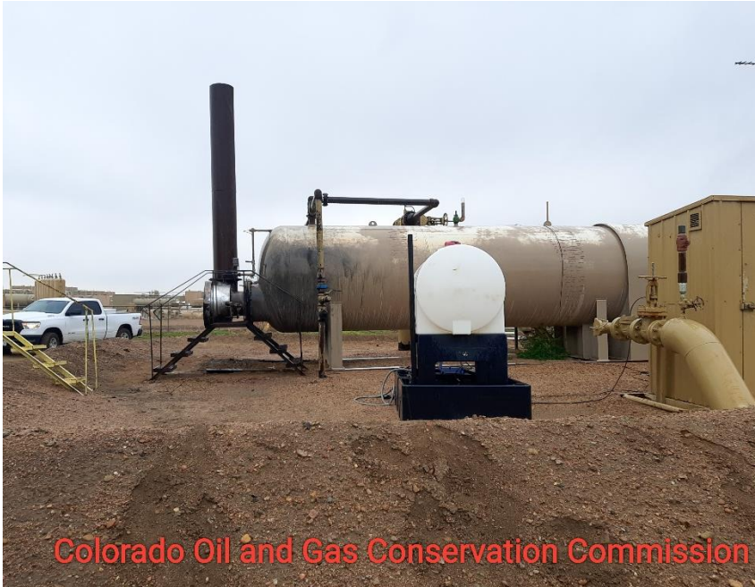
Photo 3 HOZ sep fire damage
