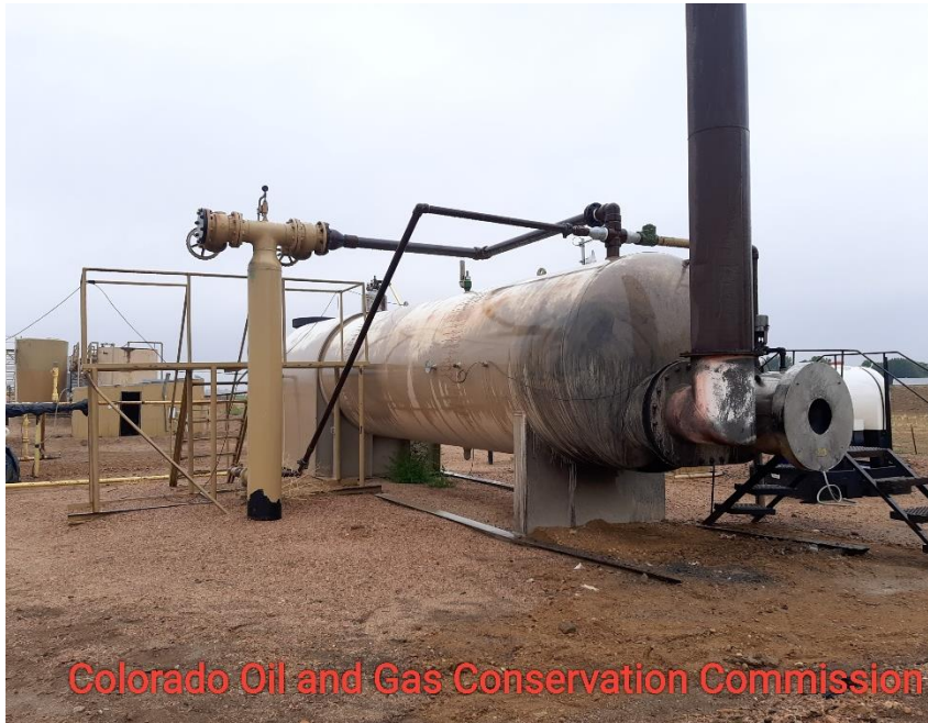
Photo 1 HOZ sep fire damage
