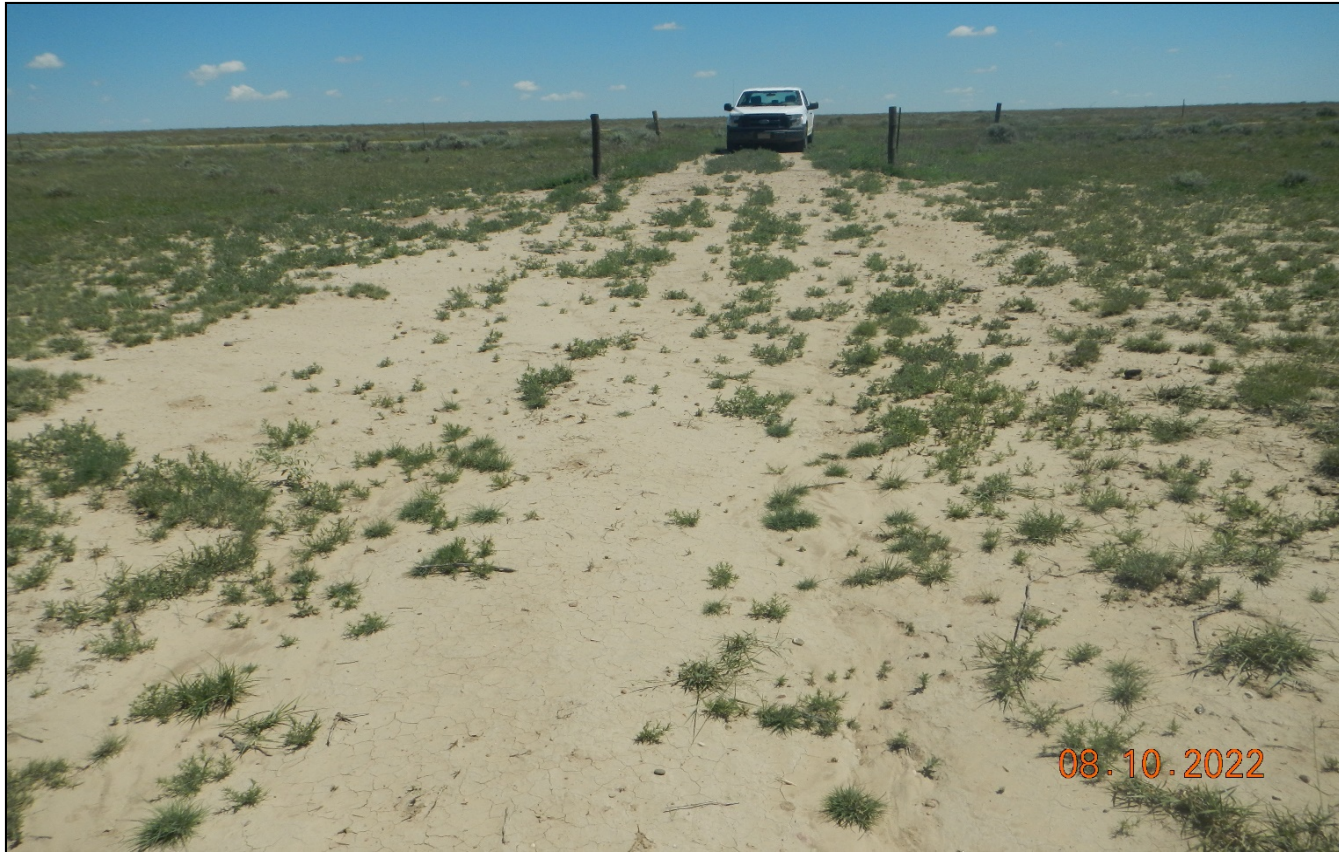
Photo 6. Facing east toward the entrance of the access road. This area needs to be decompacted and reclaimed.
