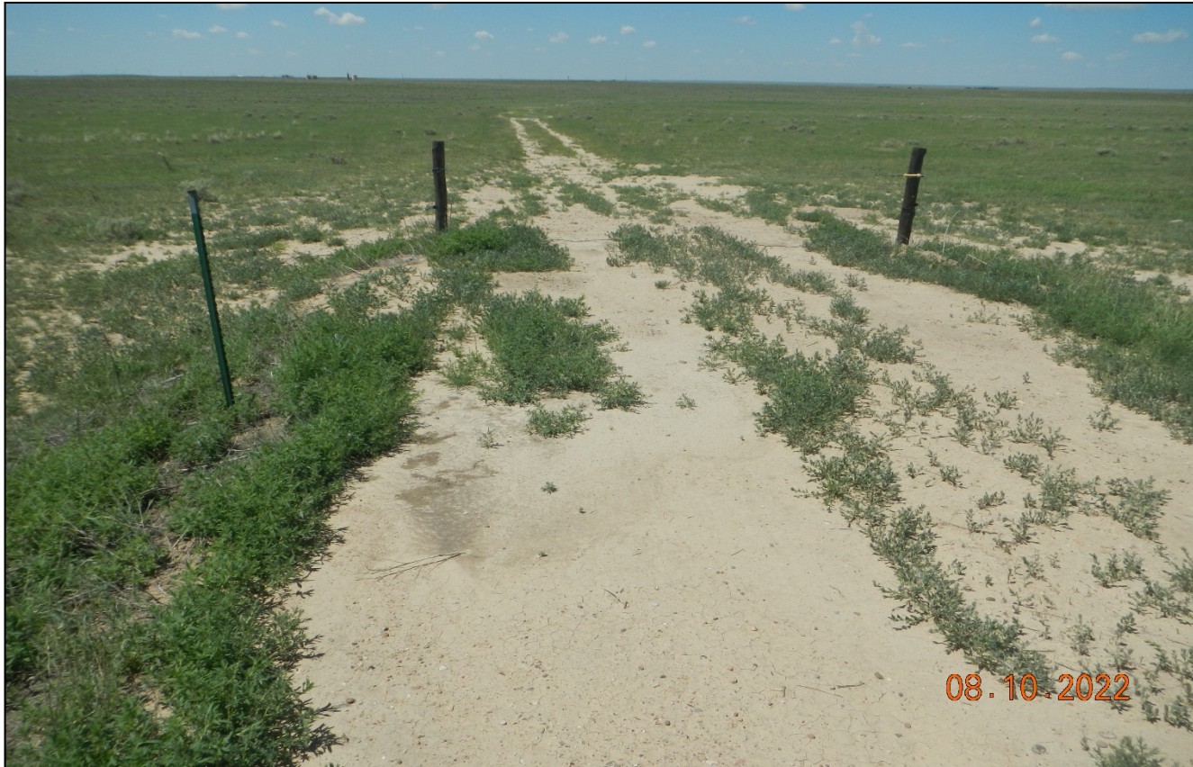
Photo 1. Facing west at the beginning of the access road. This area has not been recontoured and reclaimed. The fence needs to be put back to original boundary.
