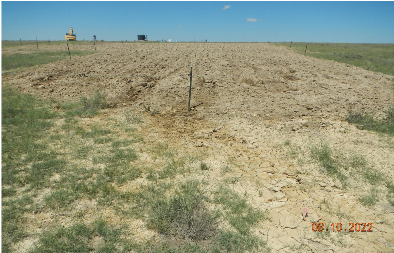
Photo 7. Facing west at the east side of the location. There are no down gradient stormwater controls to prevent sediment from moving offsite. Soils are also elevated in this area.
