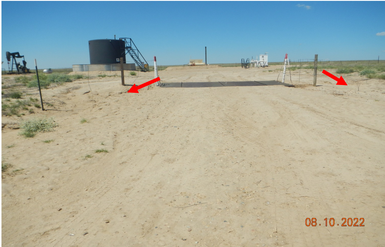
Photo 2. Facing west toward the location. Areas of erosion have been repaired. Areas along the roadside shown at red arrow need to be stabilized and seeded.
