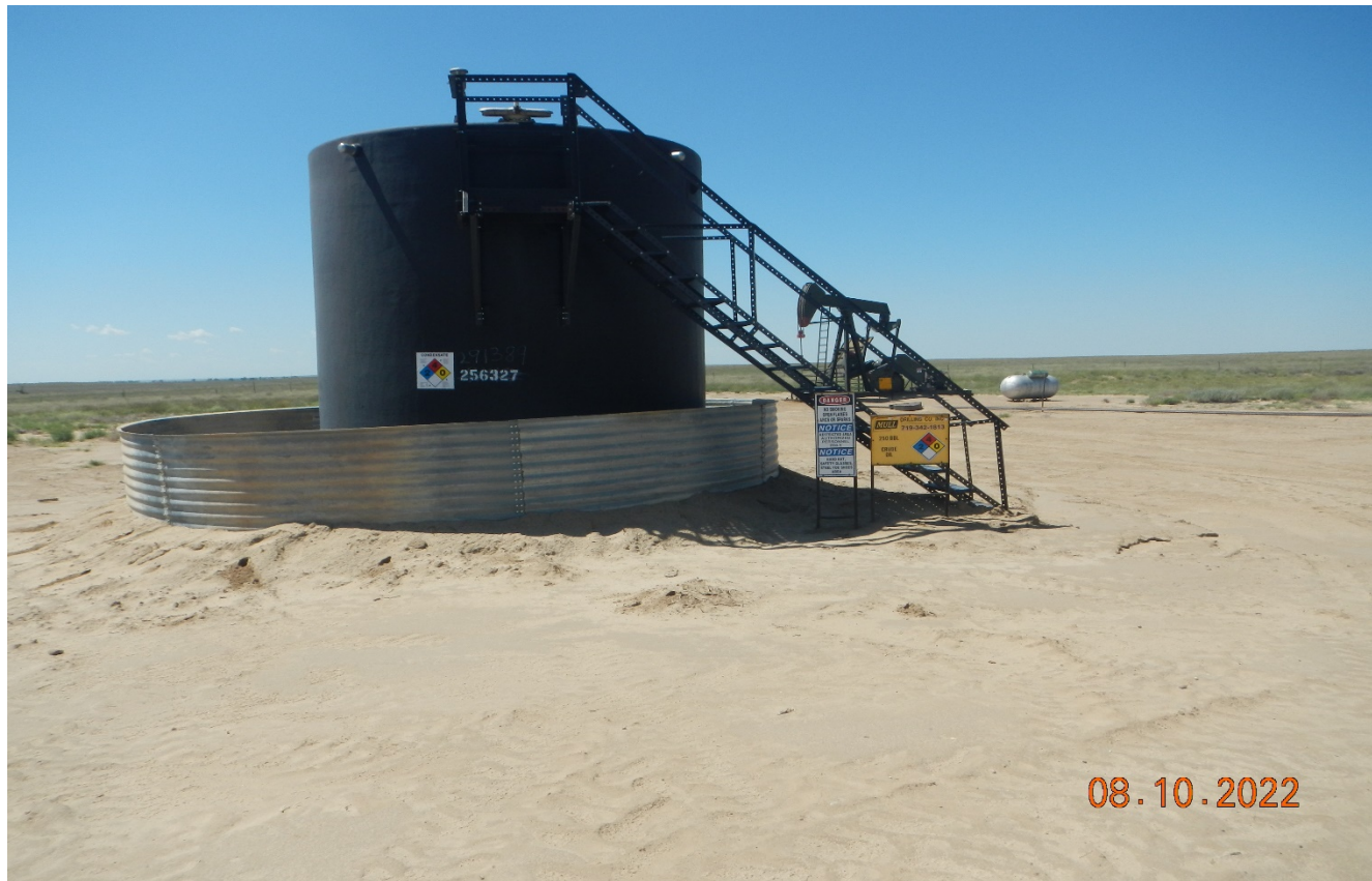
Photo 3. Facing toward the tank battery. A metal containment has been installed.
