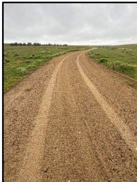
The Road had gravels added and was re-graded
